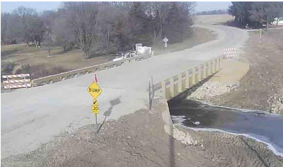
Figure 17. Composite timber bridge, Buchanan County, Iowa
