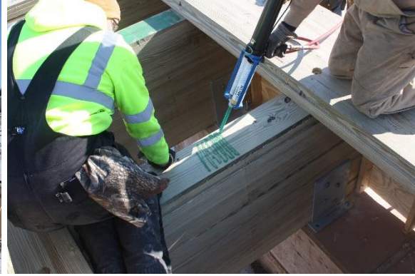
(b) Placing epoxy on tops of girders
