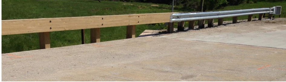
Figure 11. Guardrail on the composite timber bridge
