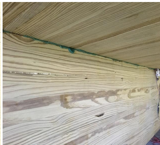
(f) Deck-girder interface after installation
