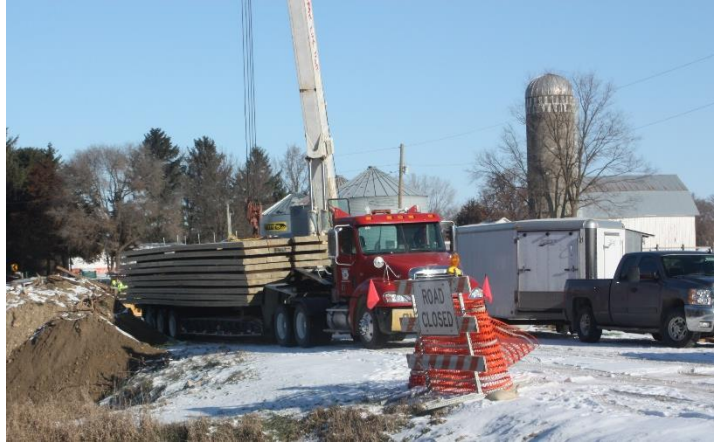
Figure 15. Glulam deck panels prior to unloading
