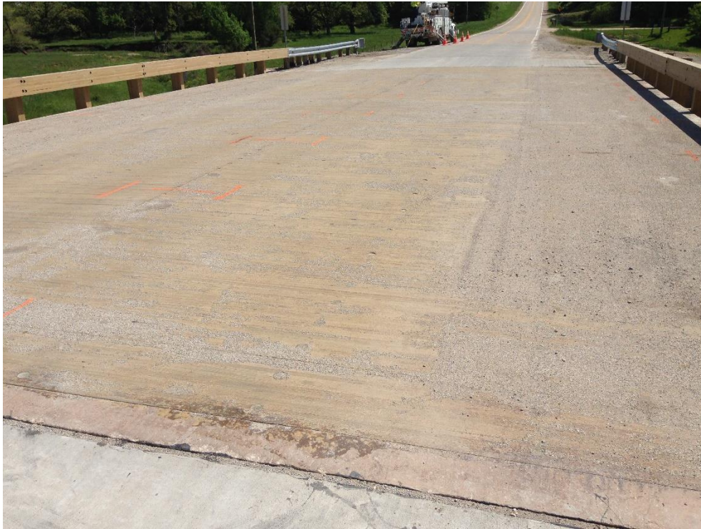
Figure 48. Epoxy wearing surface May 2015
