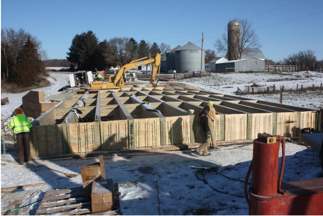
Figure 13. Girders of composite timber bridge in place
