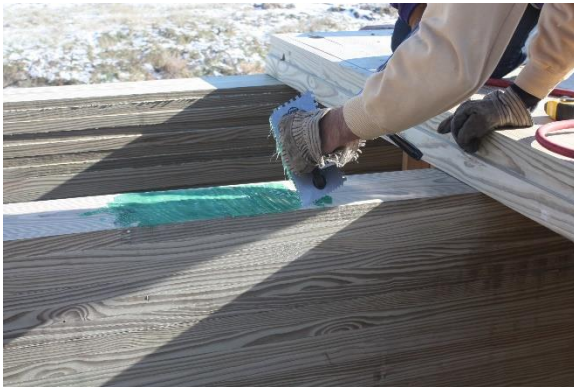
(c) Troweling epoxy with 1/4 in. v-notch trowel
