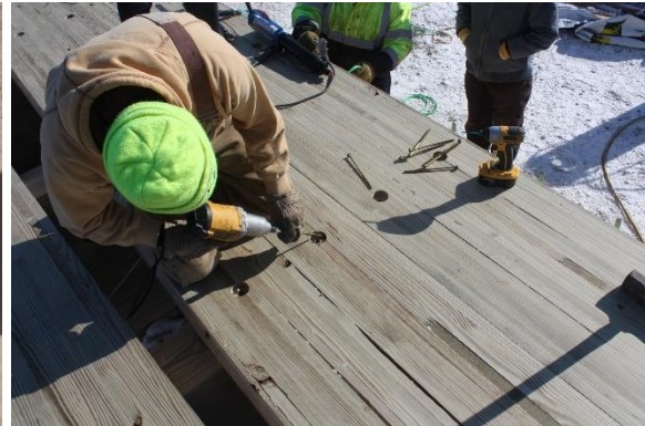
(f) Toe-nailing GRK fasteners through deck
