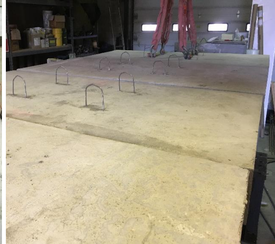
(b) Precast panels for epoxy connection
