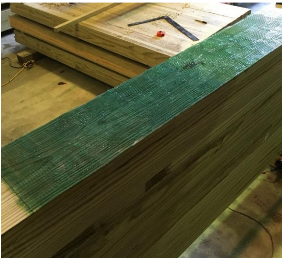
(c) Epoxy evenly spread on girder
