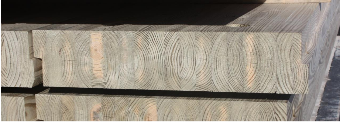
Figure 6. Lap splice edges on deck panels of the composite timber bridge
