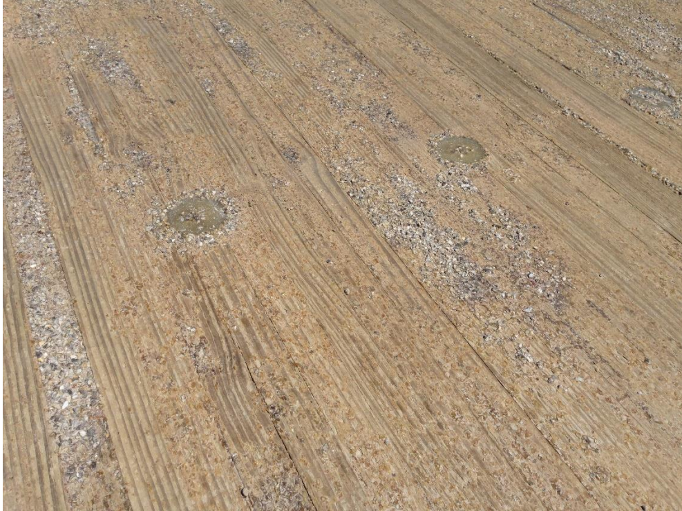
Figure 49. Epoxy filling predrilled lag screw holes
