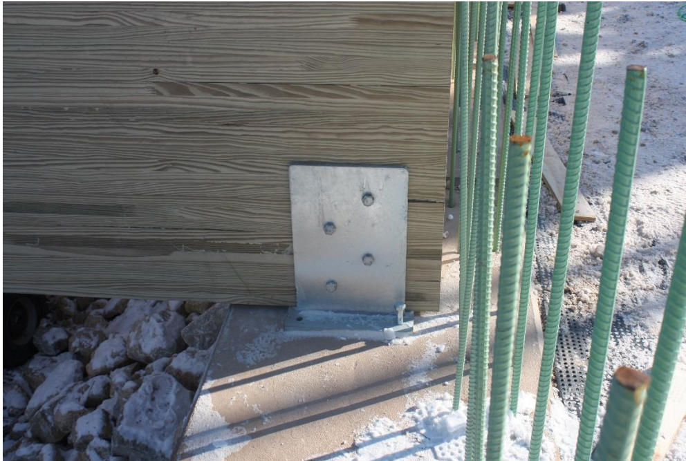
Girder anchor assembly in the field
