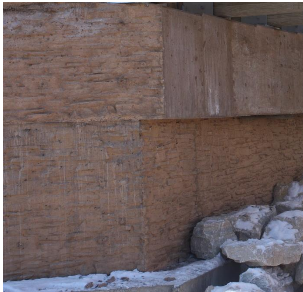
Figure 4. Composite timber bridge decorative abutment finish
