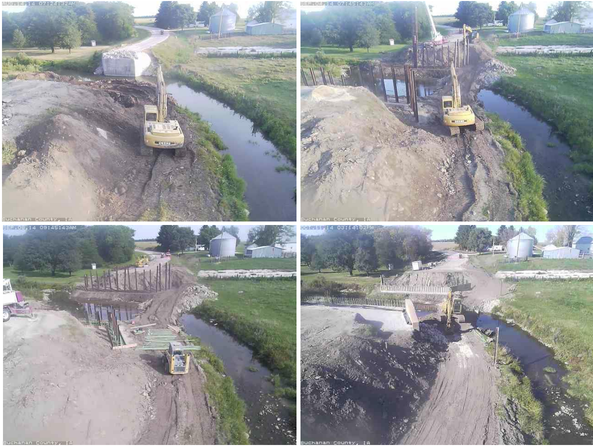
Figure 12. Composite timber bridge abutment during construction
