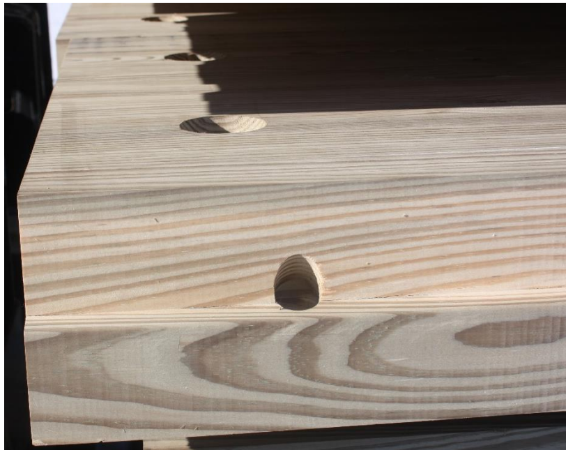
Figure 7. Predrilled holes in deck panels of the composite timber bridge
