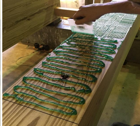
(b) 1/4 in. v-notch trowel spreading epoxy
