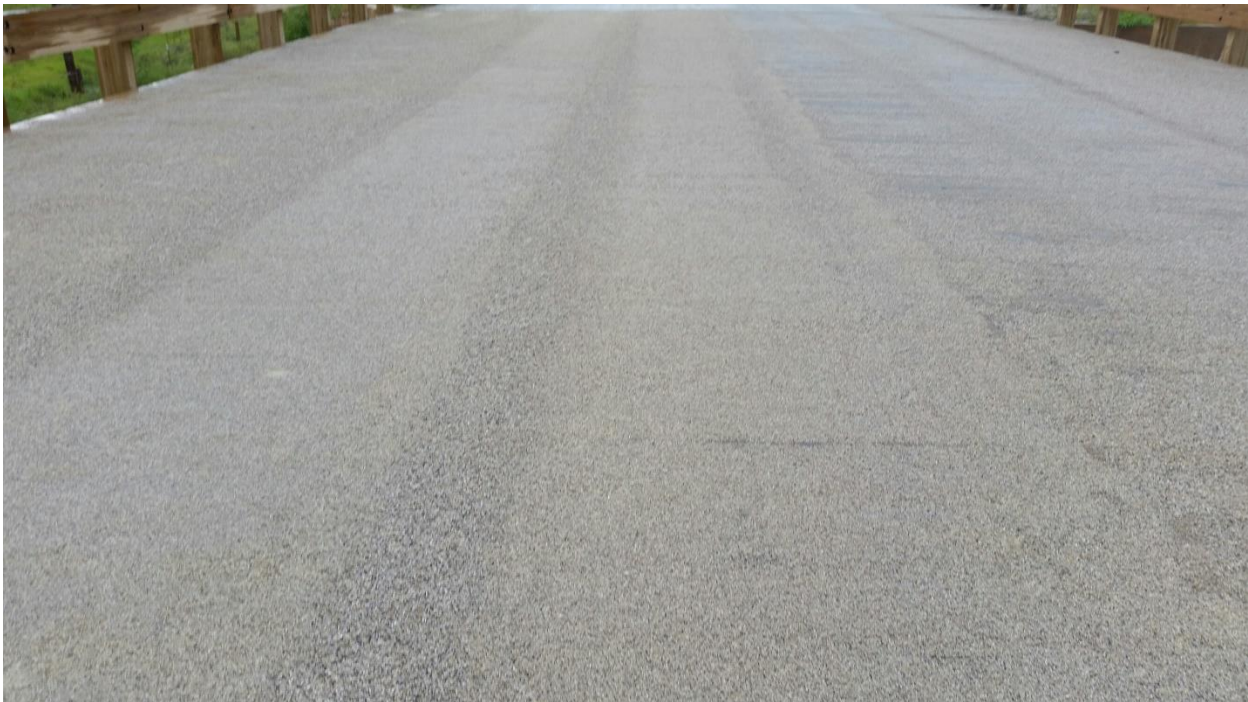
Figure 10. Epoxy chip seal wearing course on the composite timber bridge
