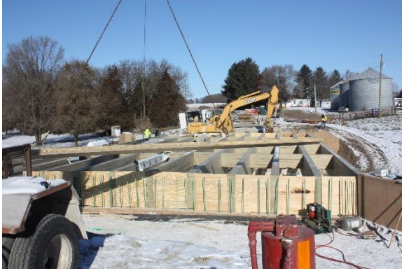
(a) Swinging deck panels
