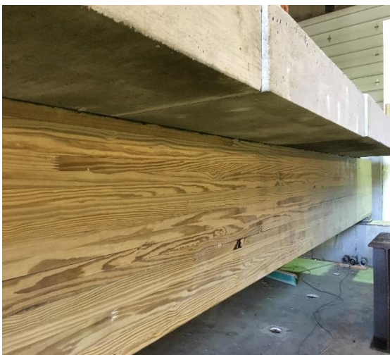
(e) Epoxyed joint btw panel and girder
