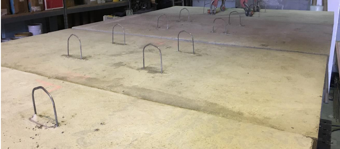
(a) Concrete deck panels without grout pockets
