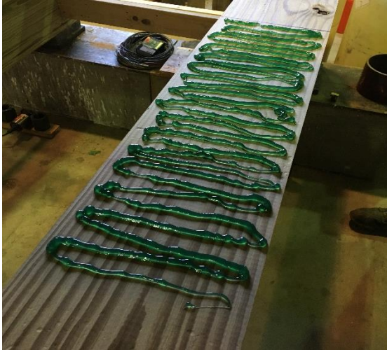
(a) Epoxy applied to girder
