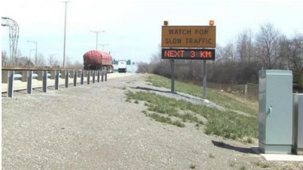
Figure 2.4 Queue warning system in Ontario, Canada (ENTERPRISE Pooled Fund Study, 2014)
