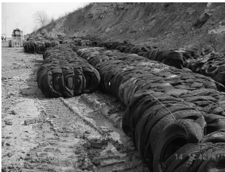
Figure 2-5 Tire bales in I-30 slope repair project, Tarrant County, Texas, 2002 (Prikryl et al. 2005)
