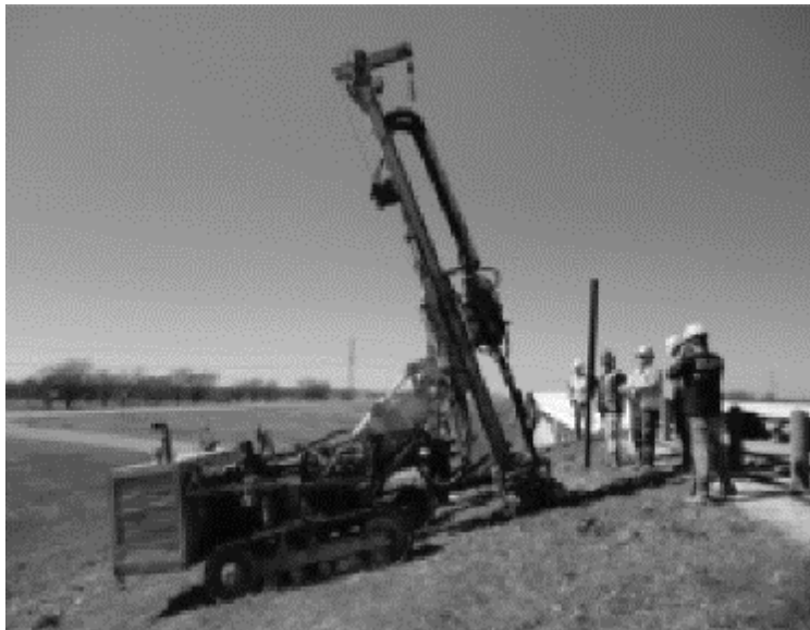
Figure 5-20 Installation of recycled plastic pins (Khan et al., 2016)
