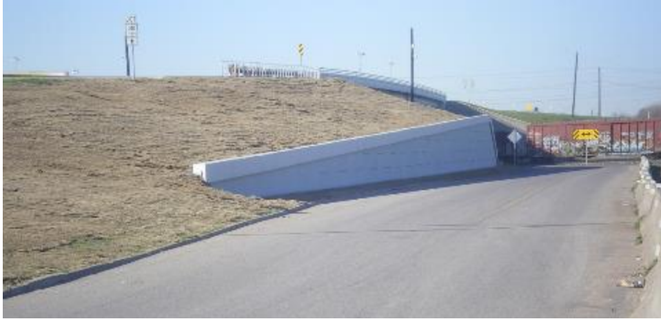
Figure 5-25 Reconstructed slope (photo courtesy of Nicasio Lozano)
