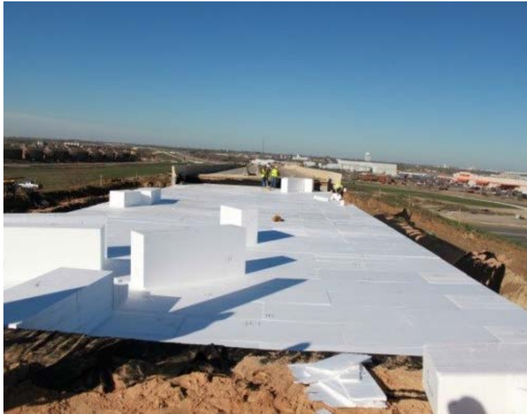
Figure 2-9 Application of gefoam in the US 67 bridge over SH 174 project (Ruttanaporamakul 2016)
