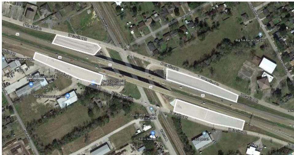
Figure 5-1 Slope failures in Jefferson County on US 69 at TX-93 Spur
