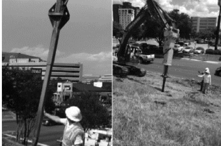
Figure 5-14 Installation of recycled plastic pins on Mockingbird slope (Hossain et al. 2017)
