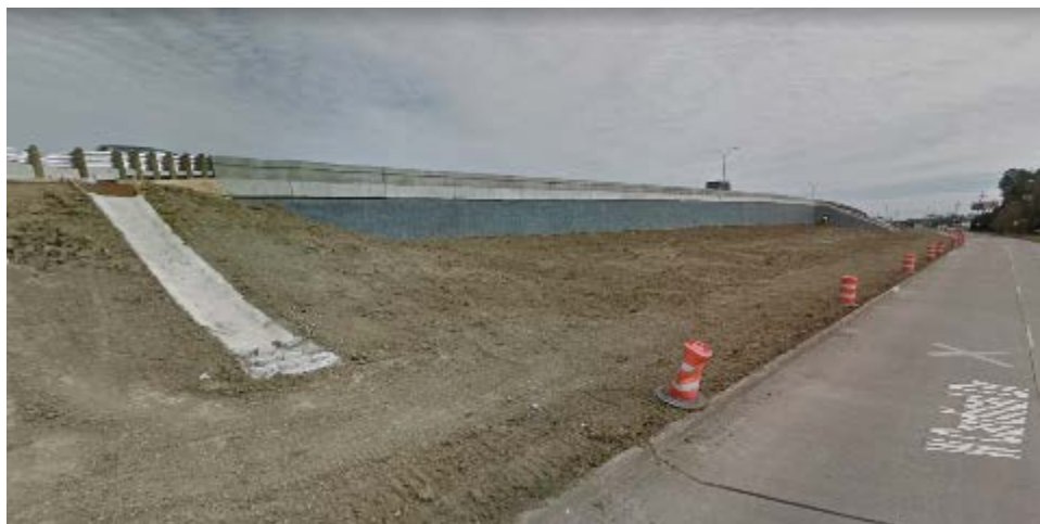
Figure 5-3 Reconstructed slope on North US 69 at TX-93 Spur
