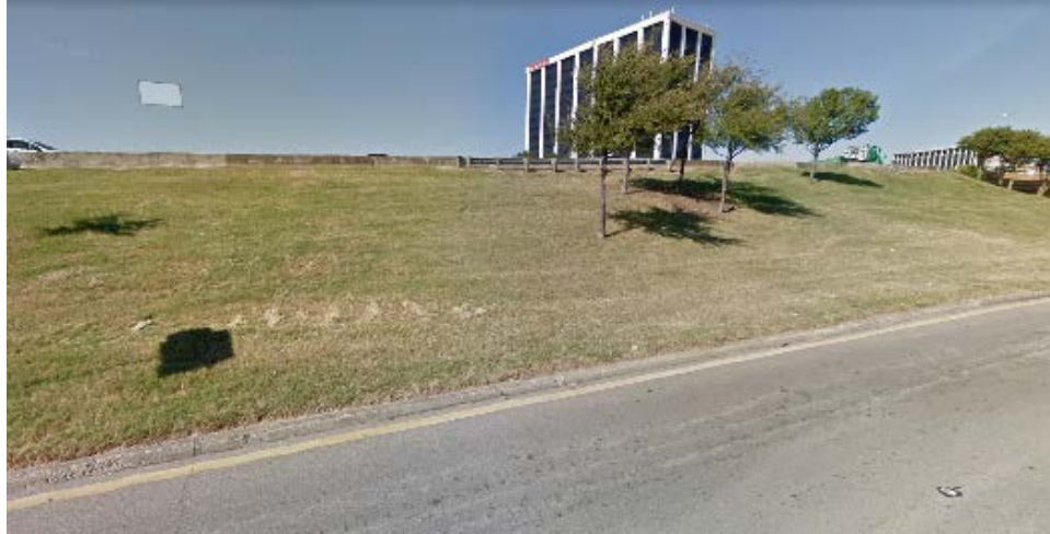
Figure 5-16 Mockingbird slope three years after stabilization with recycled plastic pins
