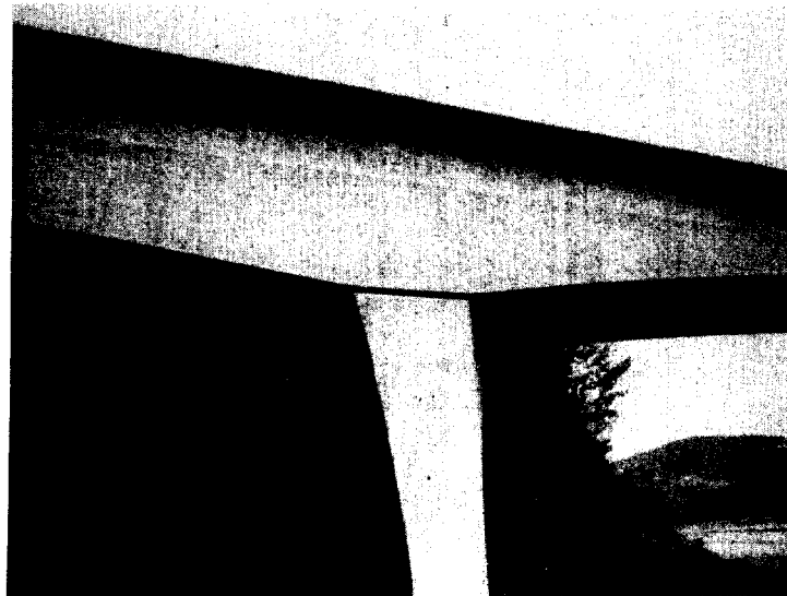
Figure 8. Closeup of bridge shown in figure 10 showing no signs of distress in spite of differential settlement of abutment.
