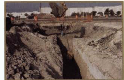
Central Texas Turnpike Construction Project.
