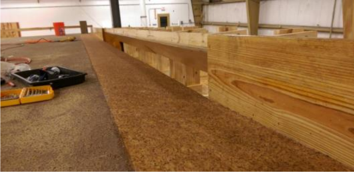
Figure 15: Completed full-scale model of conventional 15 foot curb inlet without internal slab supports.
