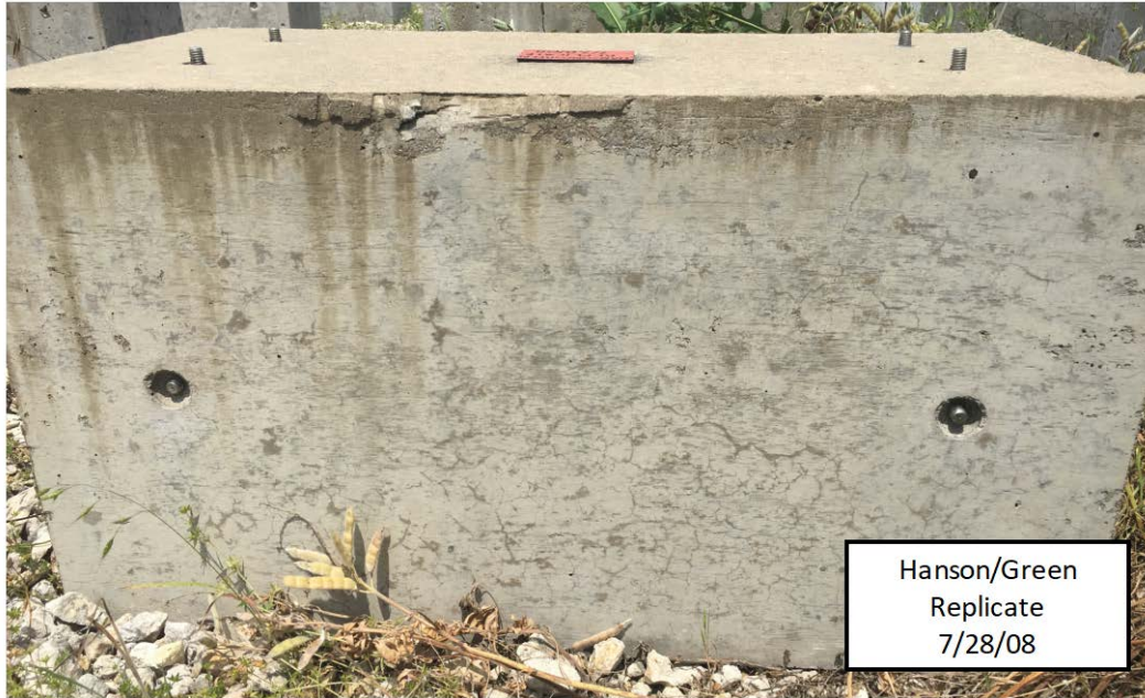
Figure 2-3: Precast plant straight cement exposure block replicate cast according to ASTM C1293 0.45 w/cm
