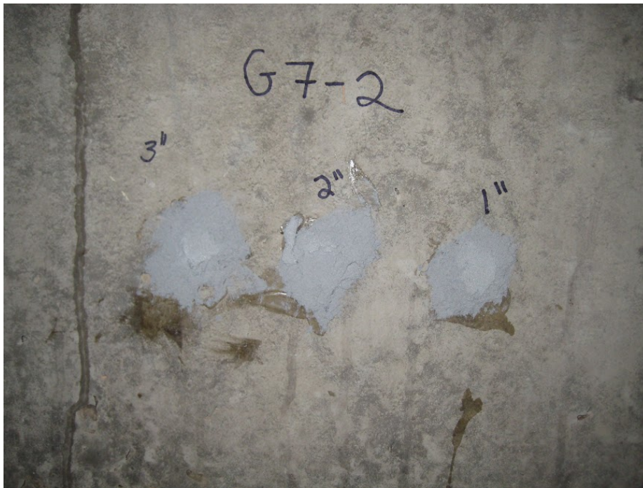
Figure 2-7: Holes sealed with cementitious grout
