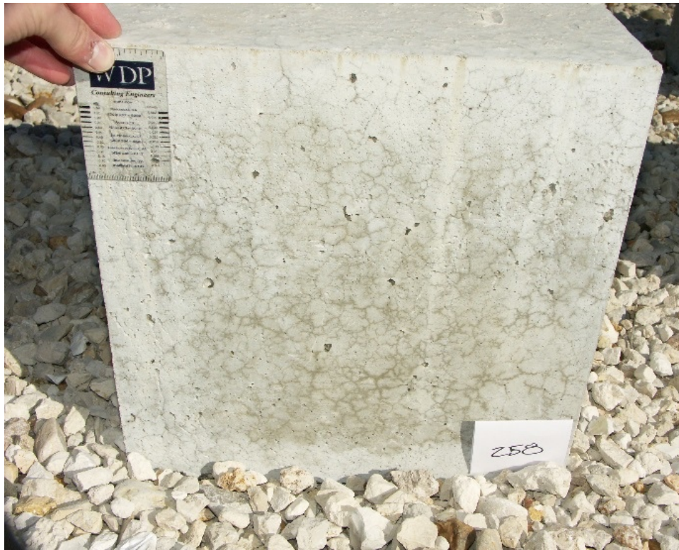
Figure 6-4: Example of Crack Rating = 3
