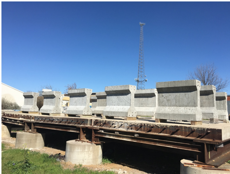
Figure 6-19: Mini girder exposure site (photo taken facing east)
