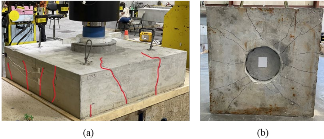
Figure B.21: Cracking after testing on (a) south-west view and (b) bottom of specimen LP-3
