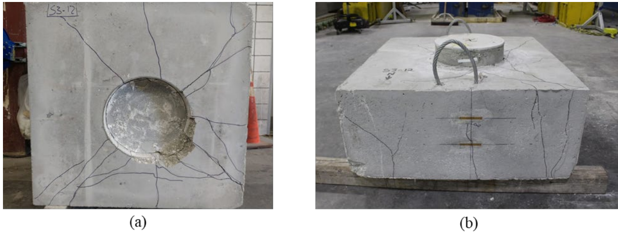
Figure A.218: Cracking after testing on (a) bottom and (b) cap of Specimen S3-12
