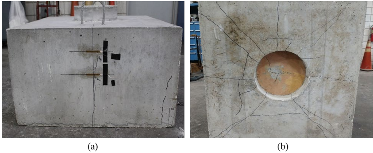
Figure A.122: Cracking on the (a) east side and (b) bottom of Specimen S2-16
