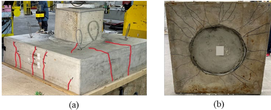
Figure B.58: Cracking on (a) cap and (b) bottom of Specimen SC-2
