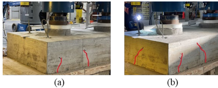
Figure B.37: Crack progression during testing at (a) 150 kips and (b) 250 kips
