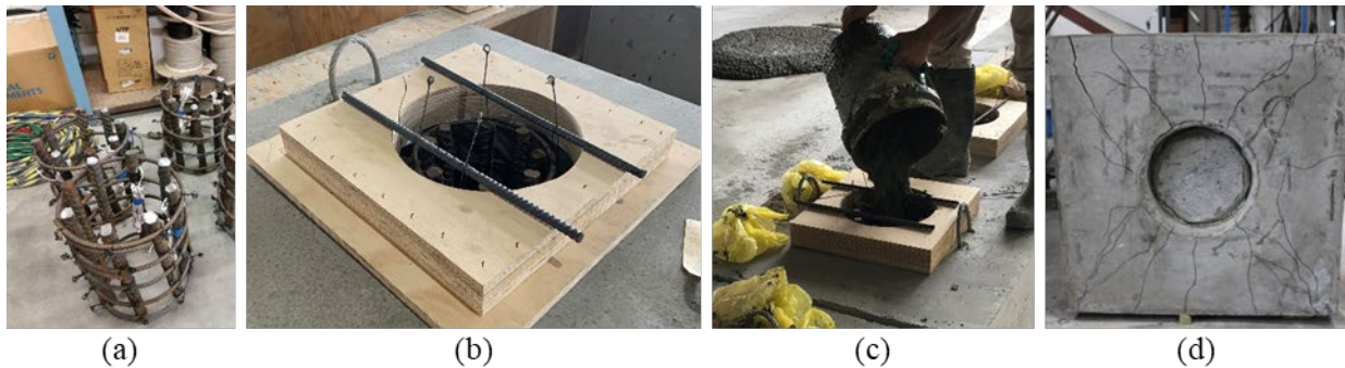
Figure 3.4: Plug construction: (a) typical plug reinforcement, (b) 3-inch cylindrical form on top of cap, (c) casting of plug concrete, and (d) 3-inch blockout on bottom of plug (after testing)
