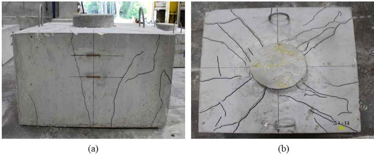
Figure A.126: Cracking on the (a) east side and (b) top of the Specimen S2-17
