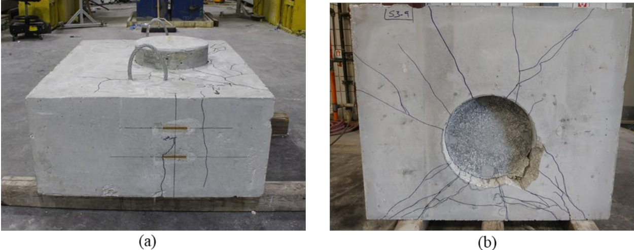
Figure A.197: Cracking on (a) cap and (b) bottom of Specimen S3-9
