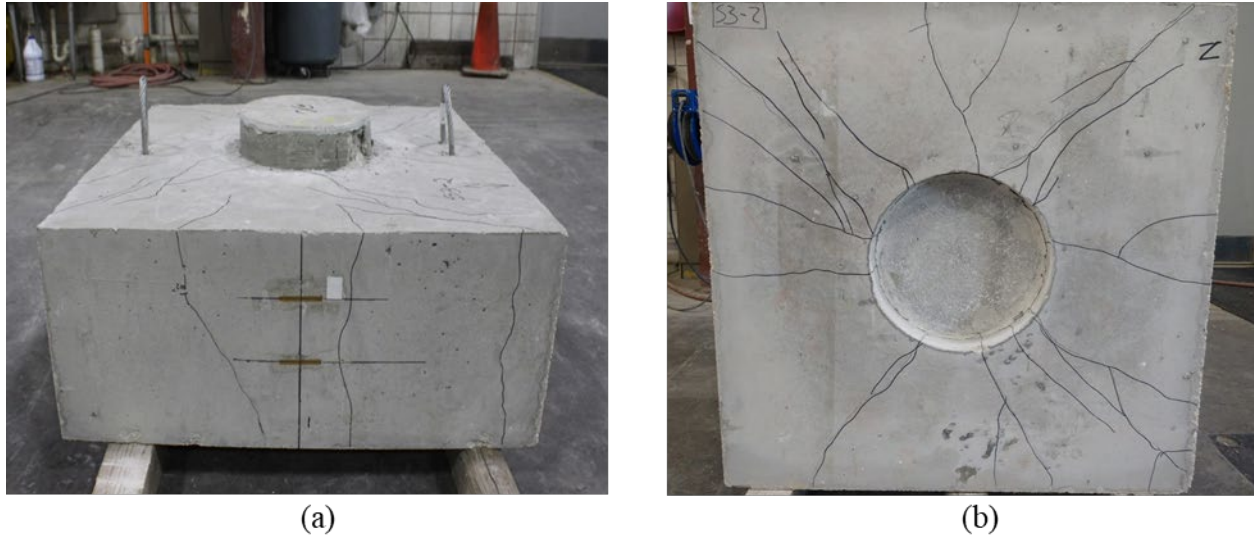
Figure A.150: Cracking after testing on (a) east side of cap and (b) bottom of Specimen S3-2
