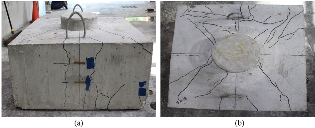
Figure A.130: Cracking on the (a) east side and (b) top of the specimen S2-18
