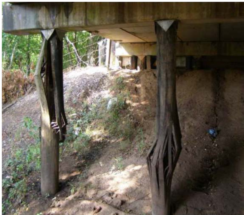
Figure 11. Bridge in District 04 with Damaged Timber Pile Substructure.
