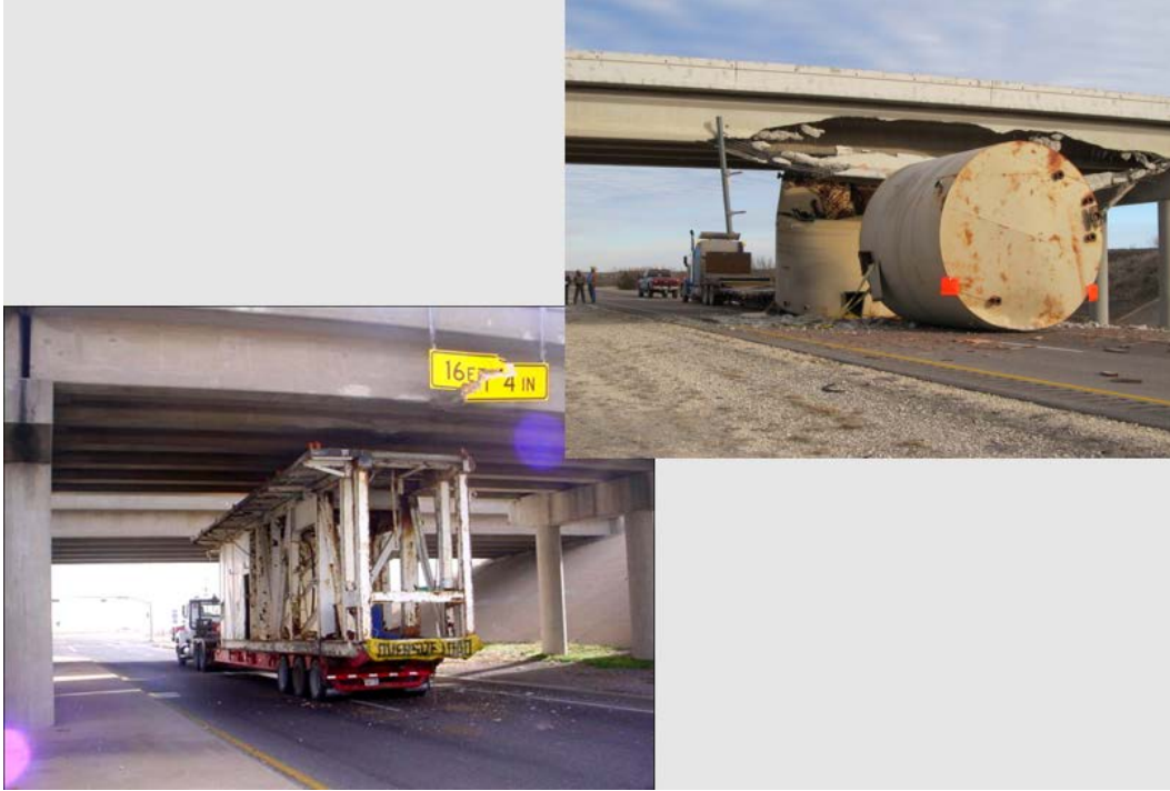
Figure 27. OS/OW Vehicles Hitting Bridges.
