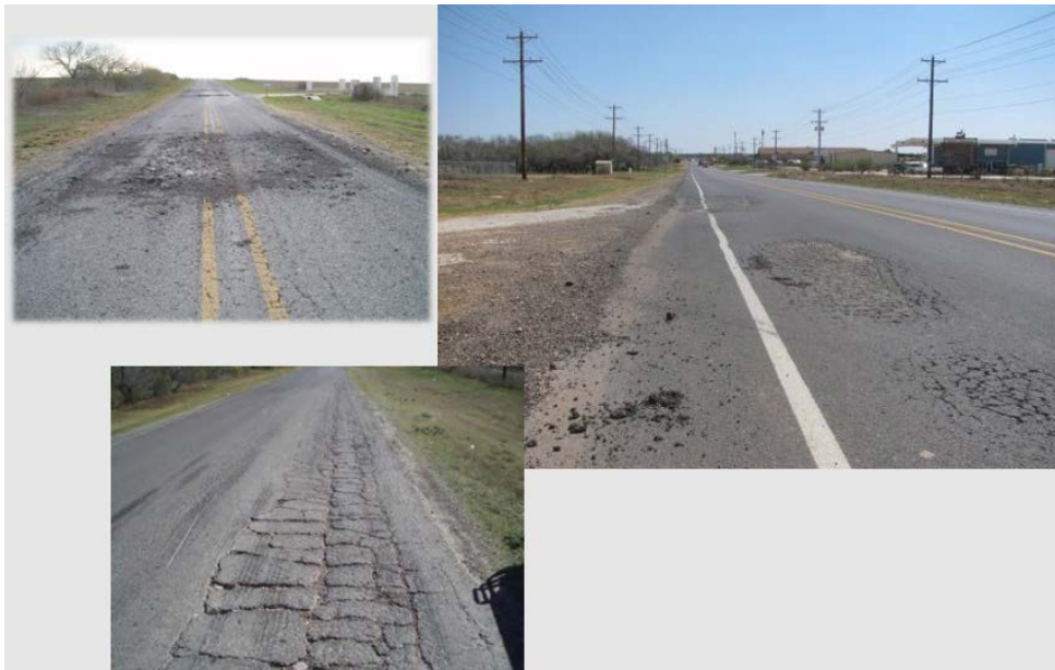
Figure 26. Roadway Damage Due to Heavy Trucks.
