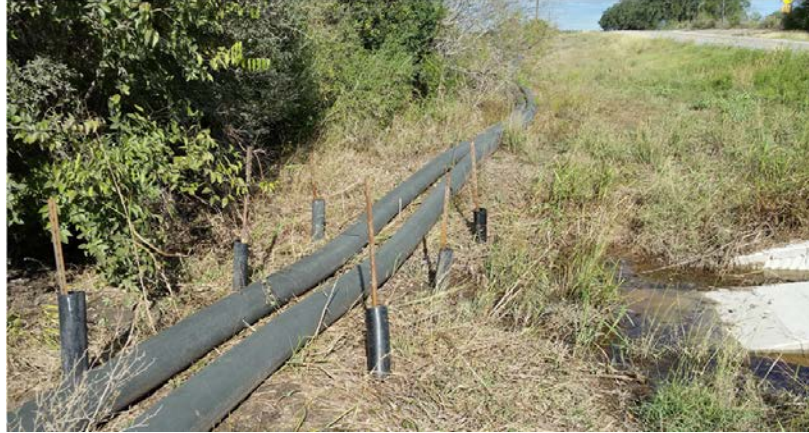
Figure 39. Example of Temporary Waterline in State Roadway Right of Way in Texas.
