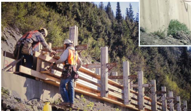
Center: Laborers drill holes in the top of existing retaining walls where vertical rebar will be epoxied into the holes. Left: Forms for the guard wall are installed on top of the retaining wall. Right: The guardwall after the forms have been removed. After final curing, the concrete will be stained to emulate the colors of stone.
