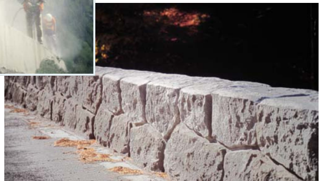
Center: Laborers drill holes in the top of existing retaining walls where vertical rebar will be epoxied into the holes. Left: Forms for the guard wall are installed on top of the retaining wall. Right: The guardwall after the forms have been removed. After final curing, the concrete will be stained to emulate the colors of stone.
