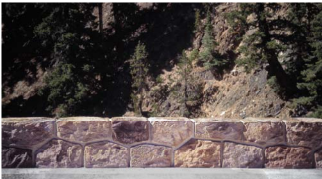
The final guardwall, after staining.
