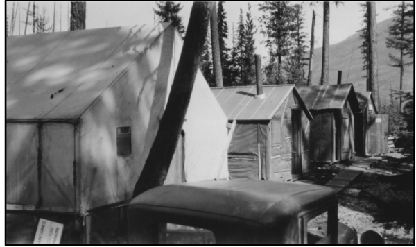
Engineering Camp at Tunnel Creek during a 1930's era reconstruction and surfacing project. Final Construction Report, Columbia Falls-Glacier Park, Section 13-F1. WFLHD Archives.
