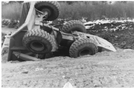
An incident on a 1961 project along the Wayan-Freedom Highway. WFLHD Archives.
