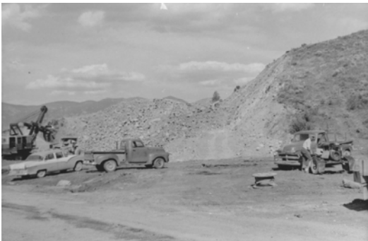
Work on the Wayan-Freedom Highway, 1961. WFLHD Archives.
