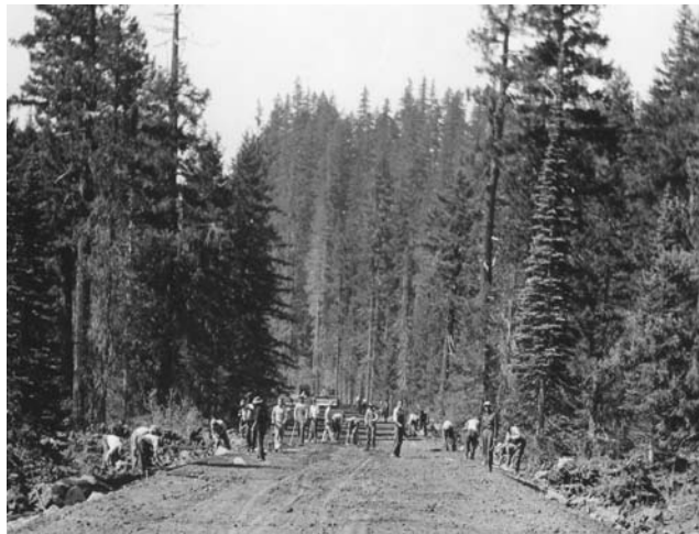
A crew of 50 men hand finishing the graded road on the Santiam Highway (Oregon Forest Highway Project NR-23-H), 1933-34. Photo from Final Construction Report, WFLHD Archives.
