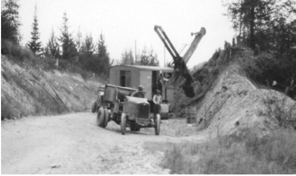
By the time Walt Langlitz went to work on the Beartooth Highway in Montana, BPR contractors had long since retired this ¾ cubic yard Northwest shovel and 2 1/3 cubic yard International truck. The photo is from a 1930's reconstruction project in Glacier National Park. WFLHD Archives.
