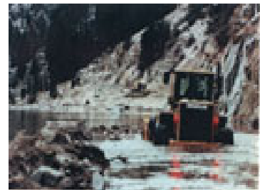
A flooded stretch of the Banks-Lowman Highway, Idaho. WFLHD Photo Archives
