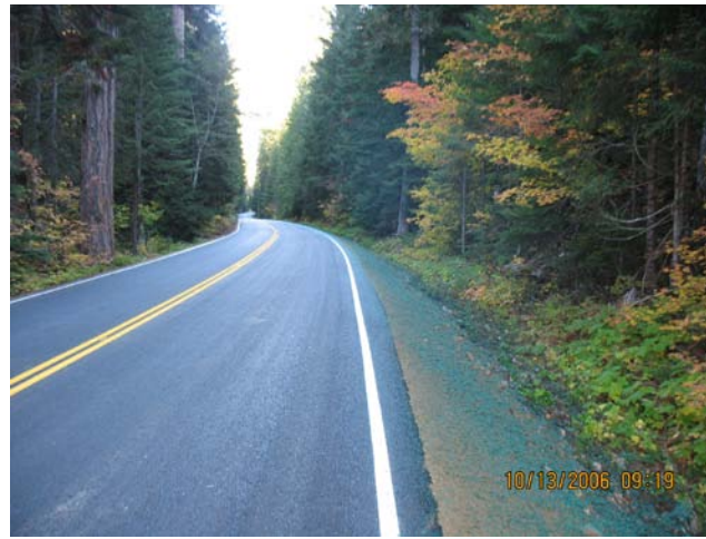
A road in Mount Rainier National Park. WFLHD Construction Archives.
