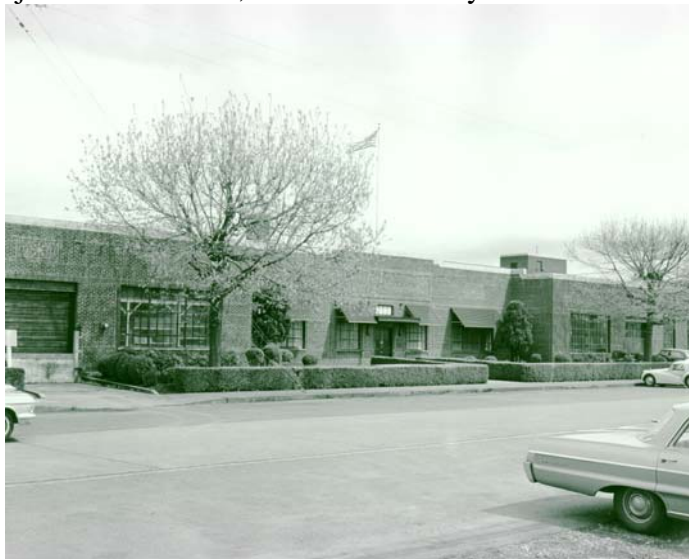
In 1965 “Building A” occupied an area that is has since become parking lot and stretched out into what is now I-5 right-of-way. The building housed the BLM maintenance shops and construction operations. WFLHD Archives.
