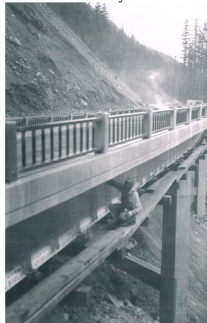
Construction on the White Pass Highway, Washington, circa 1952. Photo courtesy Ray Westby.
