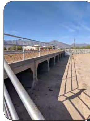
8-barrel box culvert — Pecos Road, Maricopa County, Arizona
