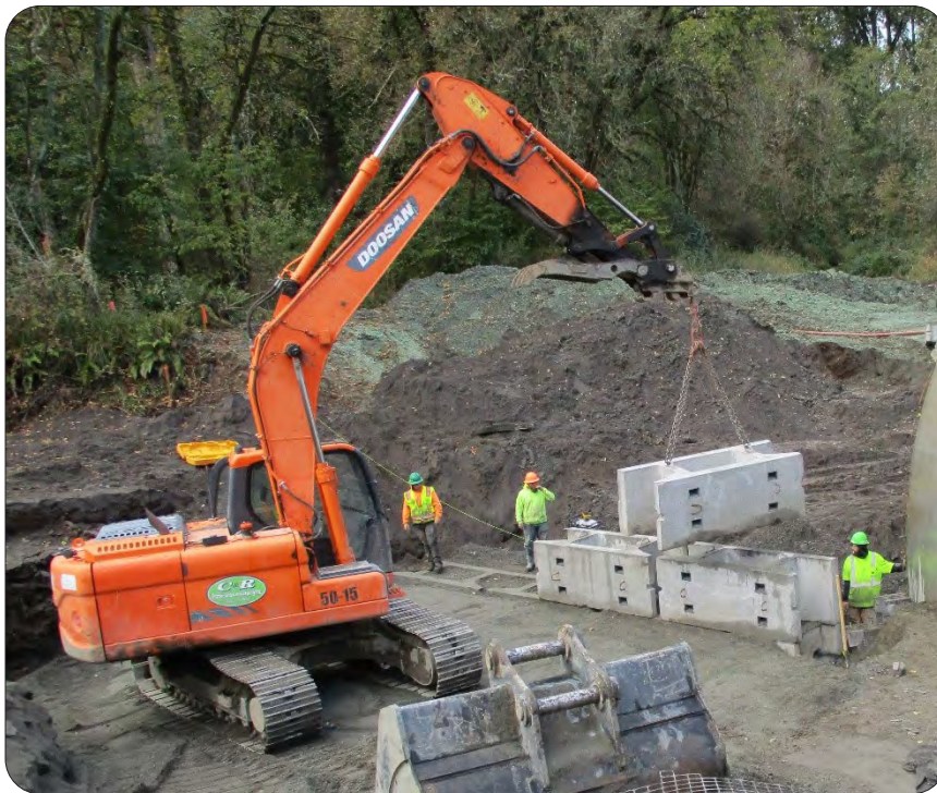
Drainage work — Gee Creek, Ridgefield National Wildlife Refuge, Washington
