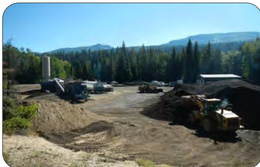
Asphalt batch plant nearby — Warren Wagon Road, Idaho
