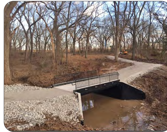
Pawnee Nation ICDBG Ceremonial Campgrounds and Nature Fit Trail Project was the 2nd to use a "Fast Cast Bridge" system and the 1st to use a "Fast Cast Bridge" system for a Pedestrian Bridge. — Pawnee, Oklahoma
