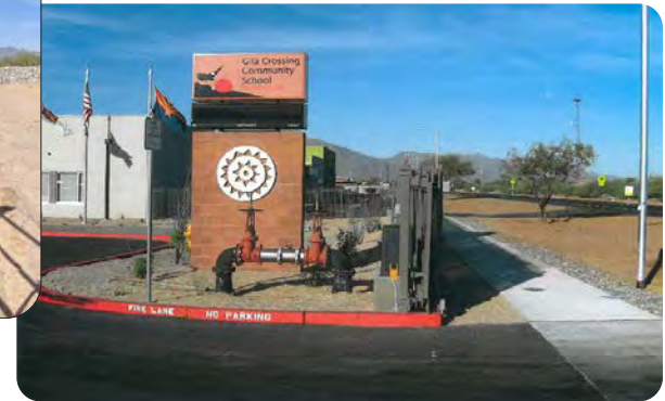
Pecos Road looking West at new Gila Crossing Community School — Maricopa County, Arizona
