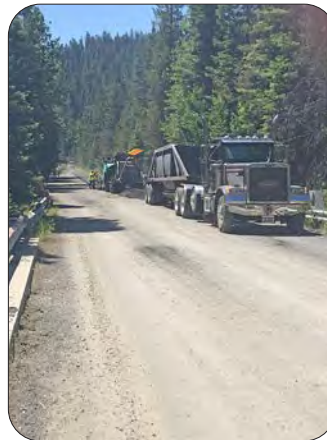
Placing the mix — Warren Wagon Road, Idaho
