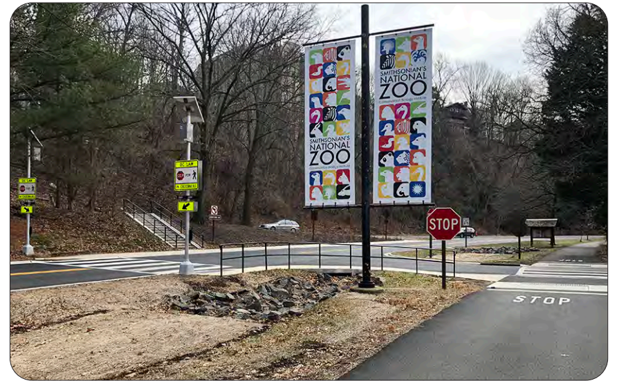
Bioretention pond and trail — Smithsonian National Zoological Park Gate, Washington, DC
