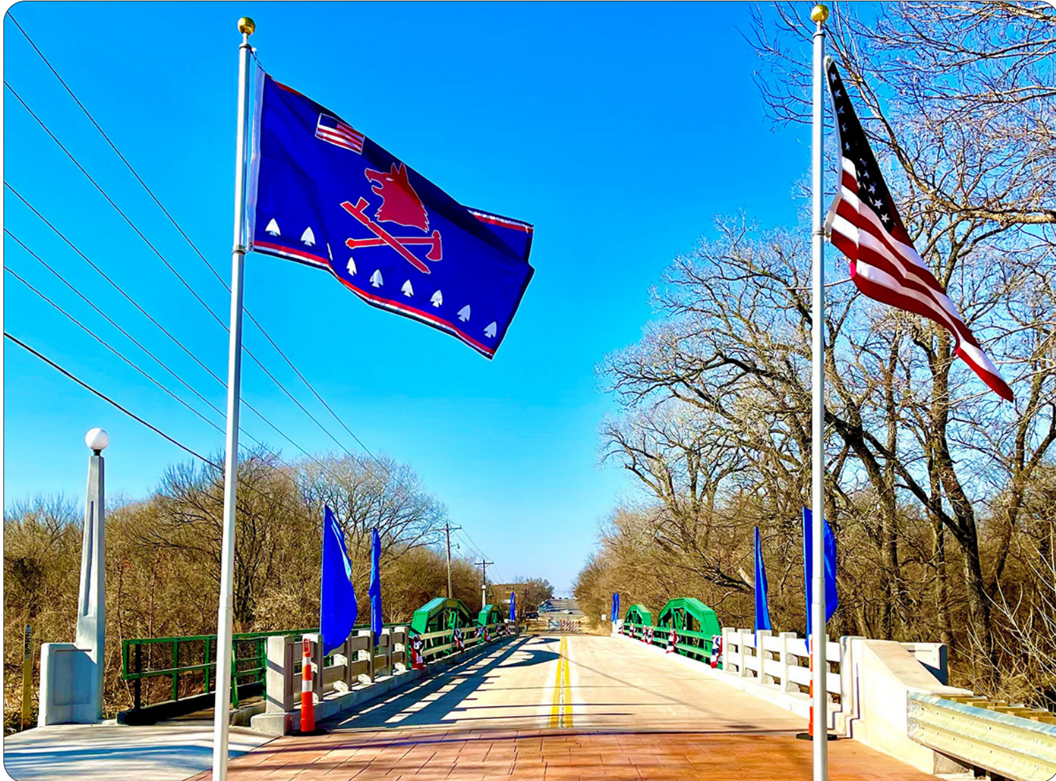
The Green Bridge, an historic pony truss bridge built in 1938, was rehabilitated by the Pawnee Nation and the City of Pawnee. Since the reopening the Pawnee Nation has received the Oklahoma ACEC Engineering Excellence Honor Award for this CM/GC Safety and Enhancement Project and are slated to receive the ACEC 2022 Engineering Excellence National Recognition Award in May 2022 as well. — Oklahoma
