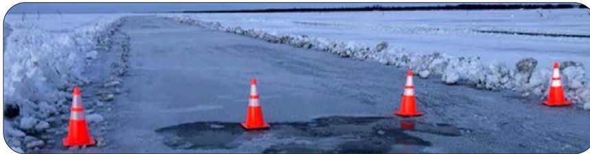
Continuous Monitoring & Maintenance is essential, here a section of the road is closed after warm weather to allow the soft surface to harden. — Alaska
