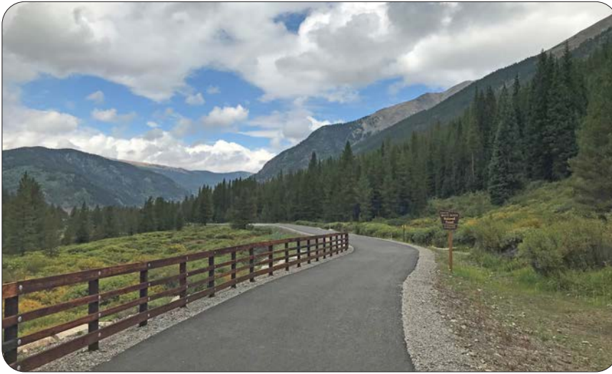
Fremont Pass Trail, Fremont Pass Recreational Pathway FLAP Project — White River National Forest, Colorado
