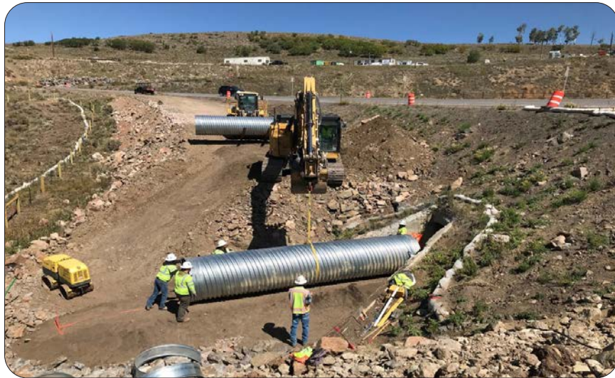
Culvert installation — Little Blue Creek Canyon, Colorado
