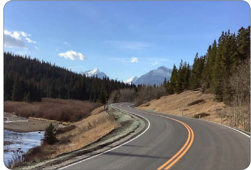
The Many Glacier Road project (above & below) rehabilitates approximately 12 miles of Many Glacier Road from Many Glacier Hotel Parking Area to the intersection in Babb, Montana on the Blackfeet Indian Reservation. In general, the project closely follows existing horizontal and vertical alignments, while providing consistent 22 foot-wide paved surfaces. The project includes improved base material beneath the roadway, new asphalt concrete pavement surfacing, replacement of failed, undersized, or otherwise deficient culverts, masonry and minor bridge work, as well as turnout and parking area reconstruction throughout project limits. — Glacier National Park, Montana
