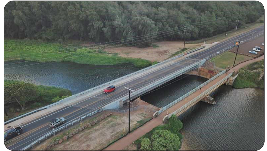
Kapaa Stream Bridge and Mailihuna Road intersection rehab and safety improvements projects (above & below) addressed bridge width, load capacity, bridge railing and transitions, and bridge approaches. The highway intersection at Mailihuna Road was also improved with lighting, signing, pavement marking, drainage, traffic signal installation, roadway widening and other improvements. — Island of Kauai, Hawaii
