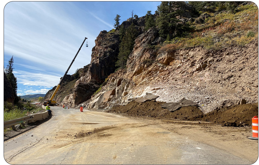
Rock Cut — Little Blue Creek Canyon, Colorado
