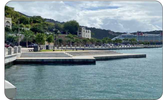
Lookout Point 2 and Dock Area — Veterans Drive Phase 1a, USVI
