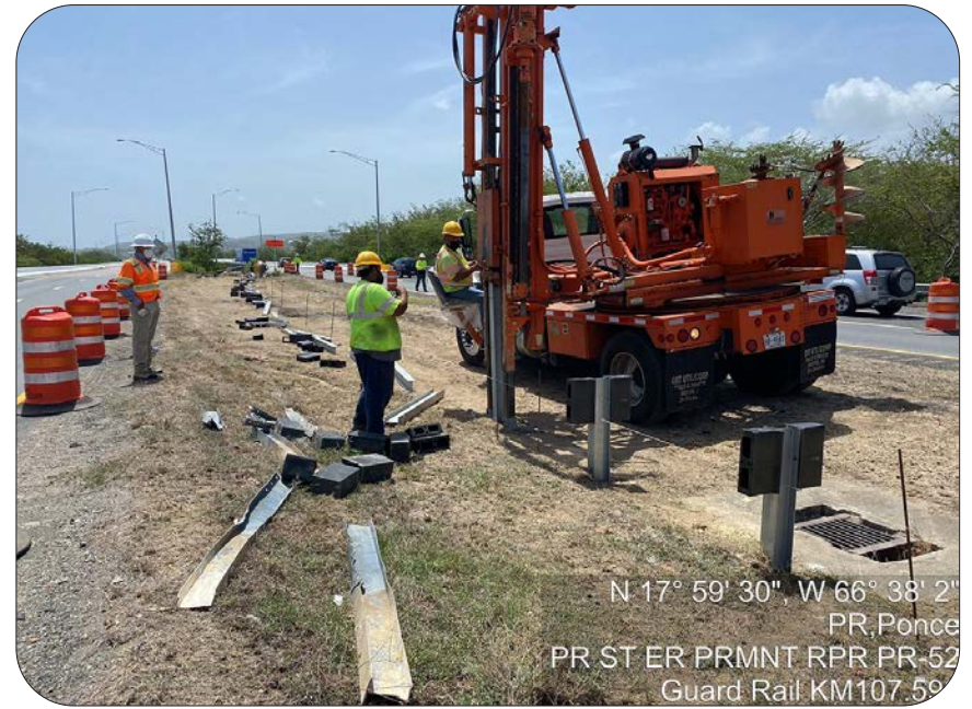
Guardrail installation (above) and (below), Jose Pabon-Rivera, EFLHD Construction Engineer inspects guardrail — Safety and signage projects, Puerto Rico
