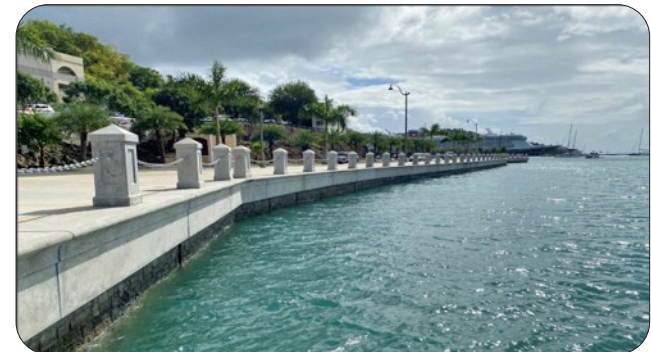
Seawall — Veterans Drive Phase 1a, USVI
