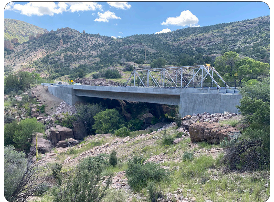
This FLAP Bridge Replacement Project addressed structural, functional inadequacies as well as the restrictive width and height limitations of two existing bridges on NM 152. The completed project provides safer and more reliable vehicular travel along NM 152, a major collector joining Interstate 25 to US 180. All photos — Gila National Forest, New Mexico.
