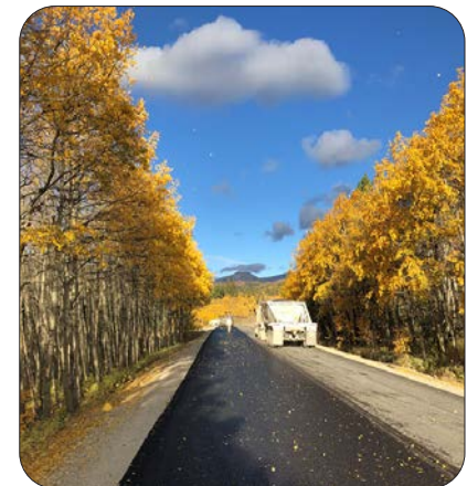
The Many Glacier Road project (above & below) rehabilitates approximately 12 miles of Many Glacier Road from Many Glacier Hotel Parking Area to the intersection in Babb, Montana on the Blackfeet Indian Reservation. In general, the project closely follows existing horizontal and vertical alignments, while providing consistent 22 foot-wide paved surfaces. The project includes improved base material beneath the roadway, new asphalt concrete pavement surfacing, replacement of failed, undersized, or otherwise deficient culverts, masonry and minor bridge work, as well as turnout and parking area reconstruction throughout project limits. — Glacier National Park, Montana
