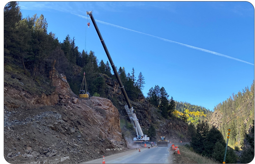
Rock Scaling — Little Blue Creek Canyon, Colorado
