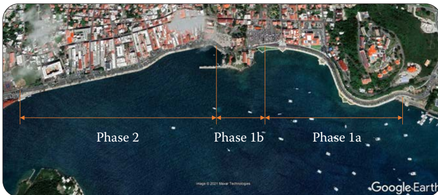
(Left) Aerial view showing project limits and work phases — Veterans Drive, USVI
