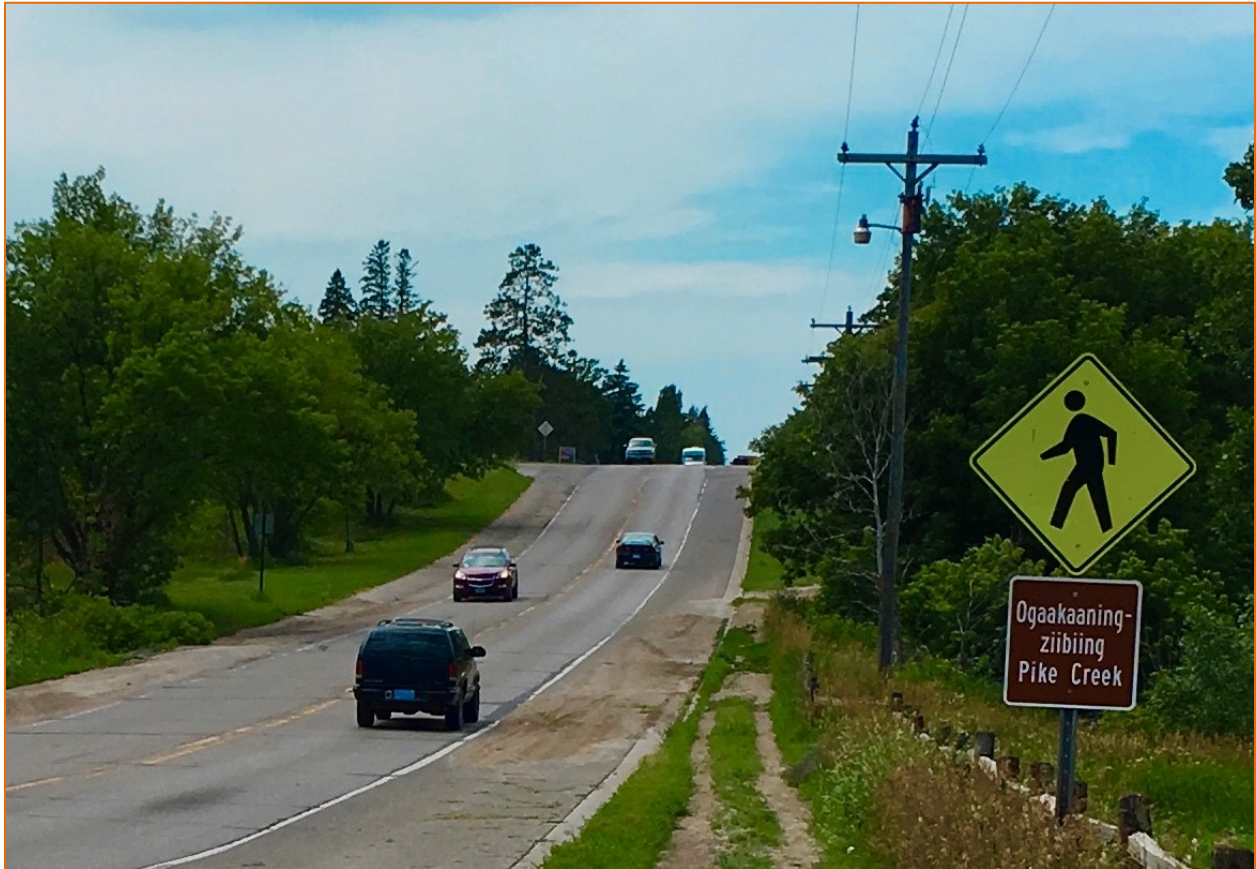
Figure 4.9 Narrow footpath in pinch point of MN-1 crossing Pike Creek
