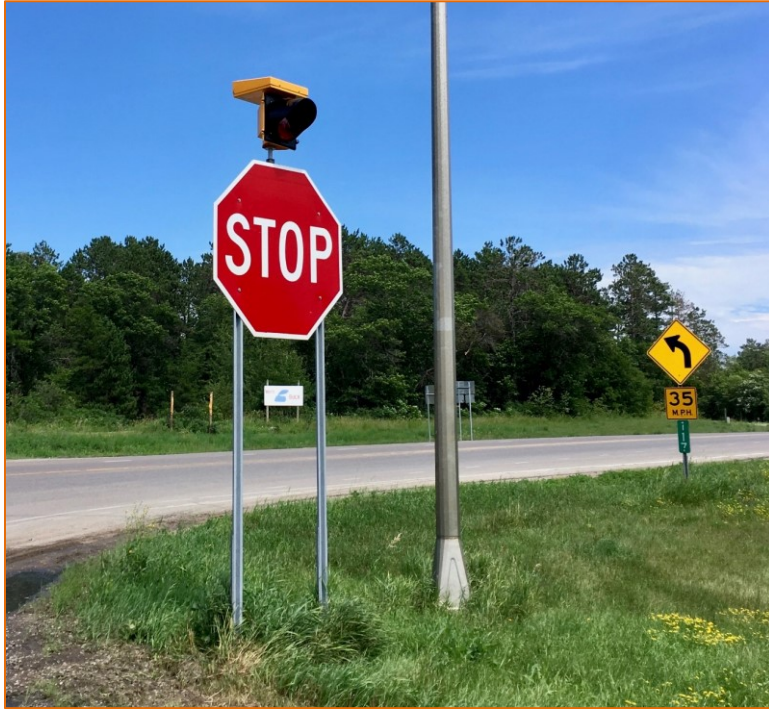
Figure 4.5 Improvements to stop sign and street lighting at MN-1 and MN-89 intersection, Red Lake
