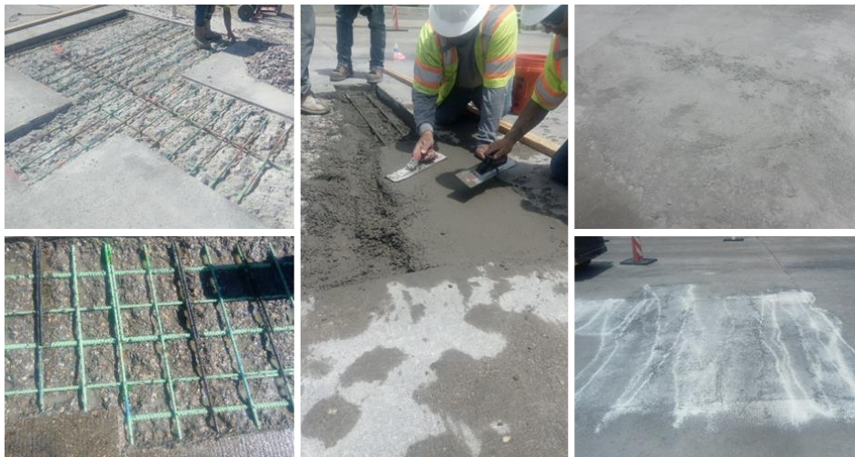
Figure 4.1 Preparation of Substrate, Pouring, Finishing, and Application of Curing Compound (P6)
