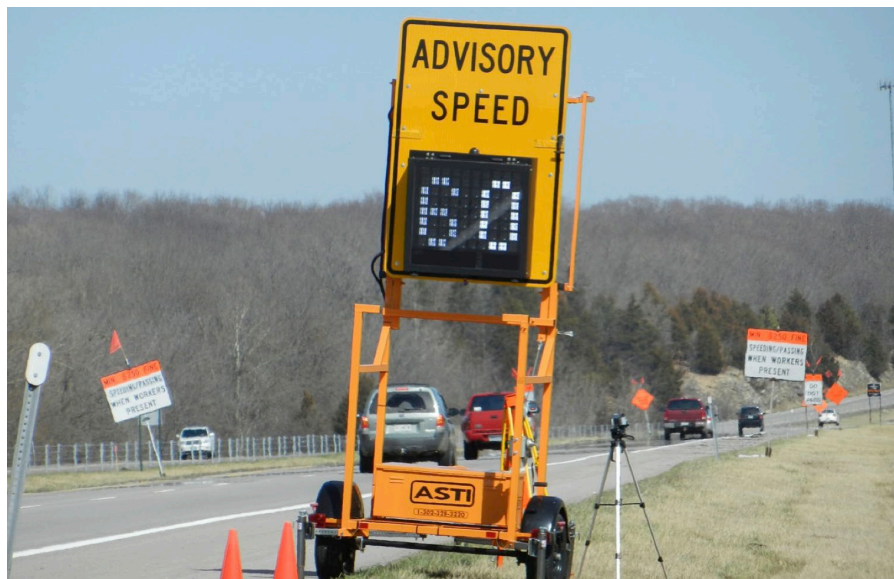
Figure 2-6. Variable Advisory Speed Limit system used in Missouri study
