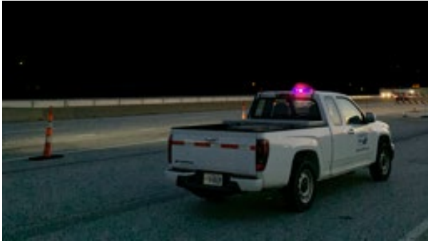
Figure 1-2. Work vehicle with flashing red and blue lights in work zone during nighttime road work on I-270 near Saint Louis, Missouri
