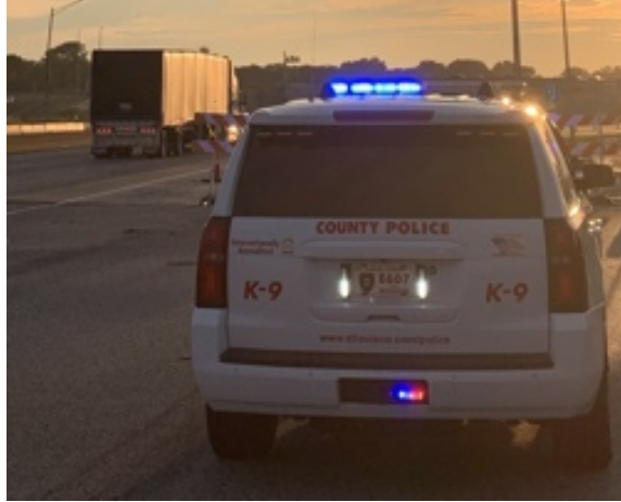
Figure 1-3. Police car parked on shoulder on work zone on I-270 near Saint Louis, Missouri
