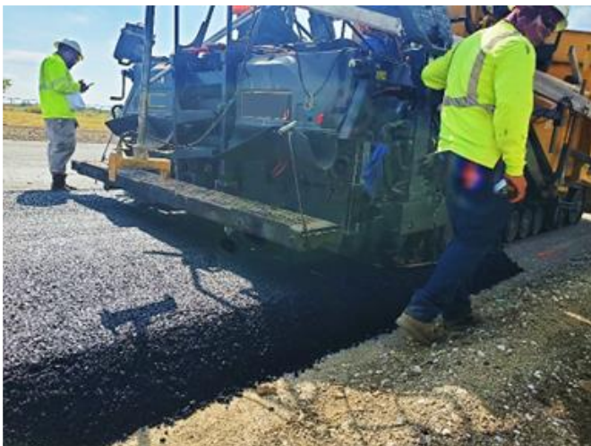
Figure 1. Thick-Lift Paving with a Tamper Bar Paver.
