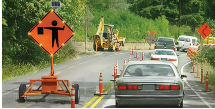
Figure 1. Example of LED Lights Outlining a Traffic Sign to Increase Driver Attention (30).
