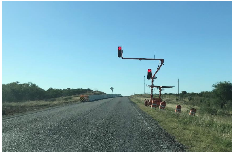
Figure 19. PTS Deployed in TxDOT Construction Work Zone.
