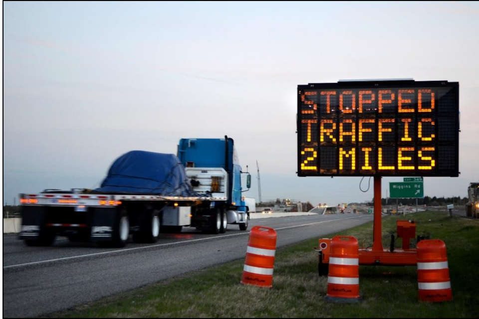
Figure 3. Example of Work Zone ITS Queue Warning Technology (47).
