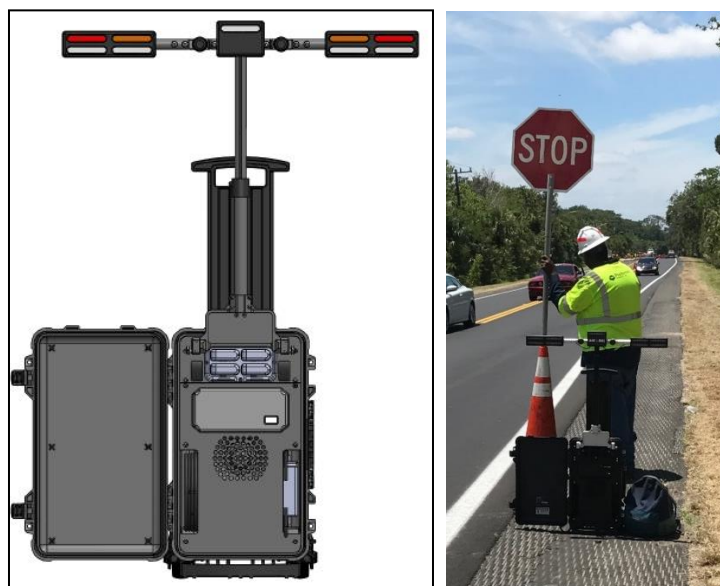
Figure 5. Visual and Audible Warning System Under Development for Flagging Operations.
