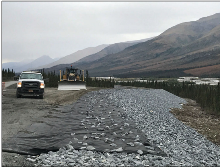
Figure 4: Geotextile Placed on top of ACE Shoulder.
