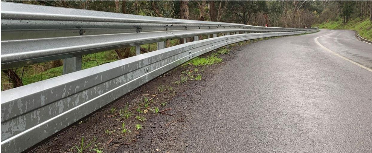
**Figure 9. Photo. Motorcycle-friendly crash barriers. Source: Safe Direction Crash Barrier Solutions.**
