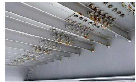
Figure 19. Splice plates and bolts
