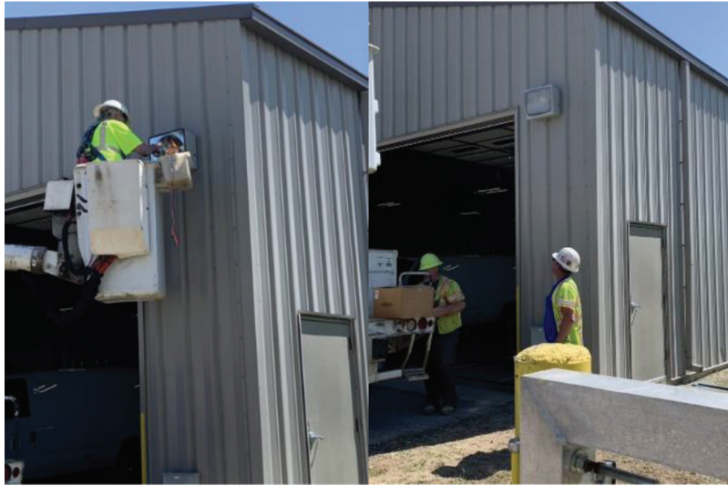
Figure 2.9 Wall luminaire installation.
