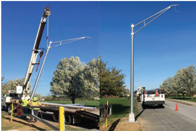
Figure 2.7 Lighting pole installation.
