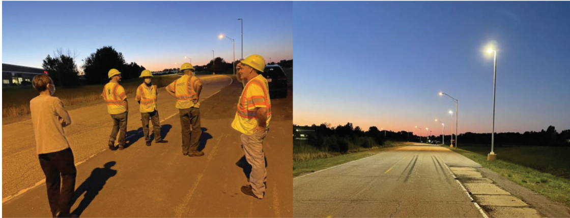
Figure 2.11 Inspection at the Indianapolis site.
