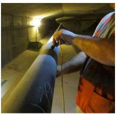
A worker begins testing on a post-tensioning tendon inside on the of the box girders that make up the Ringling Bridge.
