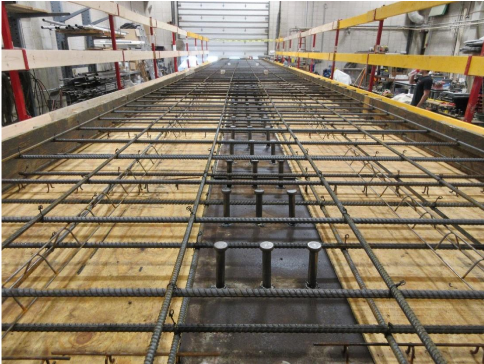
Figure 19. Composite beam shear studs
