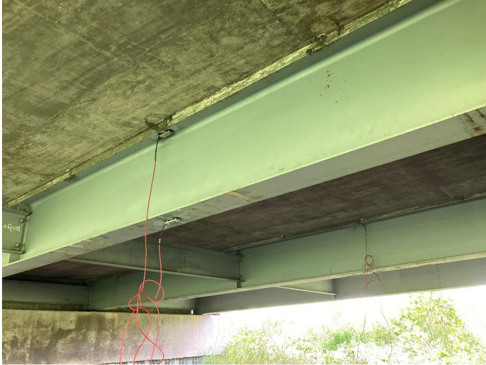
Figure 51. Strain gauges at midspan
