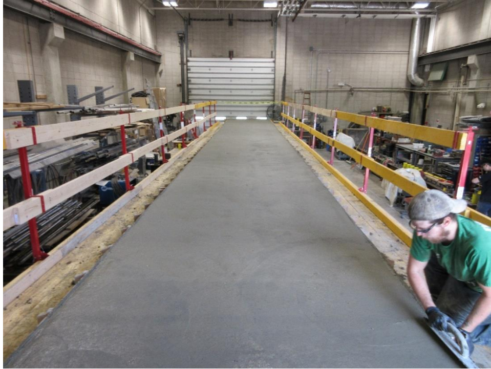
Figure 20. Composite deck concrete placement
