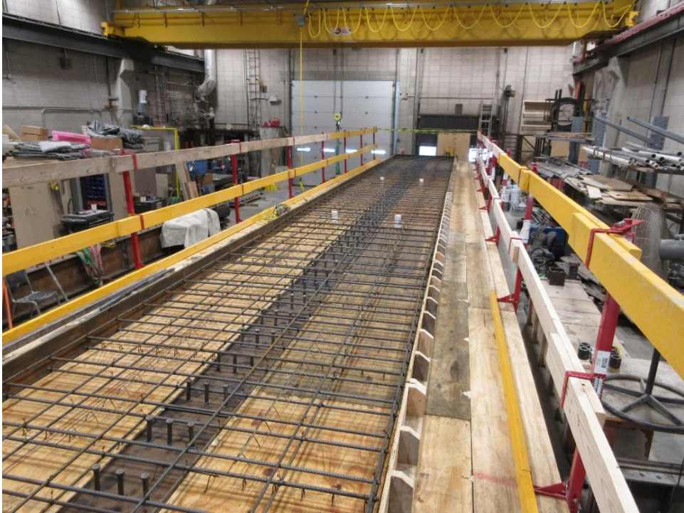
Figure 18. Composite deck reinforcement
