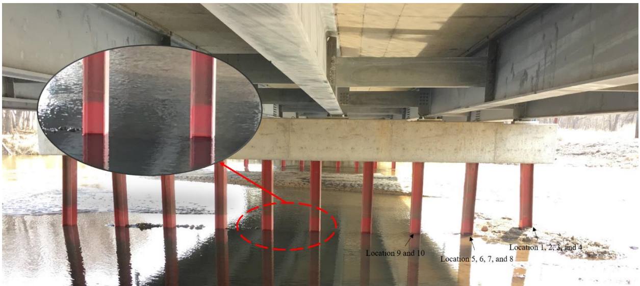
c) Galvanized and painted piles
