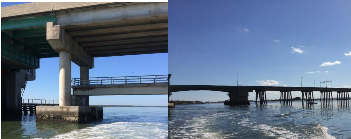
Figure 3.9. Views of Crescent Beach Bridge (Site 2).
