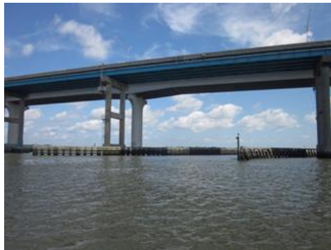
Figure 3.1. View of the State Road 312 Bridge.
