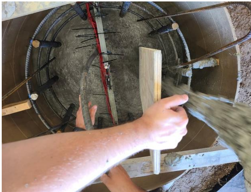
Figure 17. Photo. Plywood shield used to protect sensors during concrete placement
