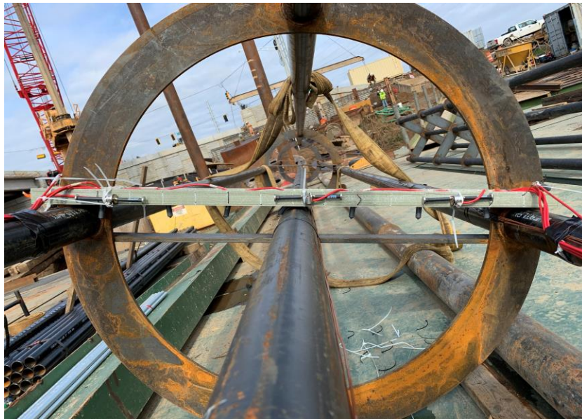
Figure 6. Photo. Sensors and FRP bar attached to the post-cooling system
