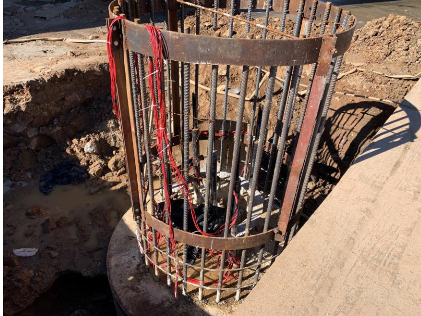
Figure 7. Photo. Cables protruding from shaft three days after placement
