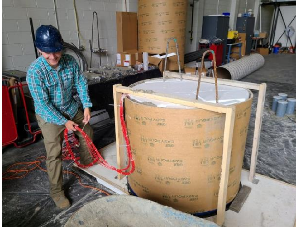
Figure 18. Photo. Test C-A-A specimen after concrete and polystyrene placement
