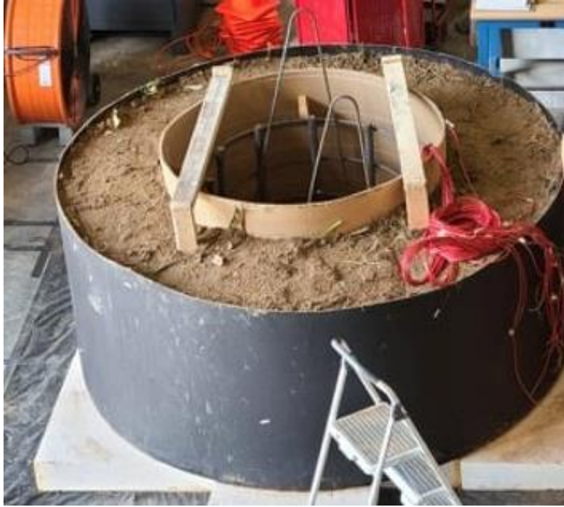
Figure 21. Photo. Test C-S-A specimen prior to concrete placement
