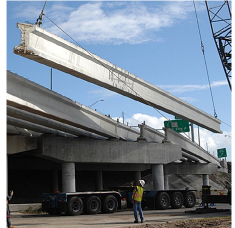
Long slender girders like this are possible because of prestressing.
