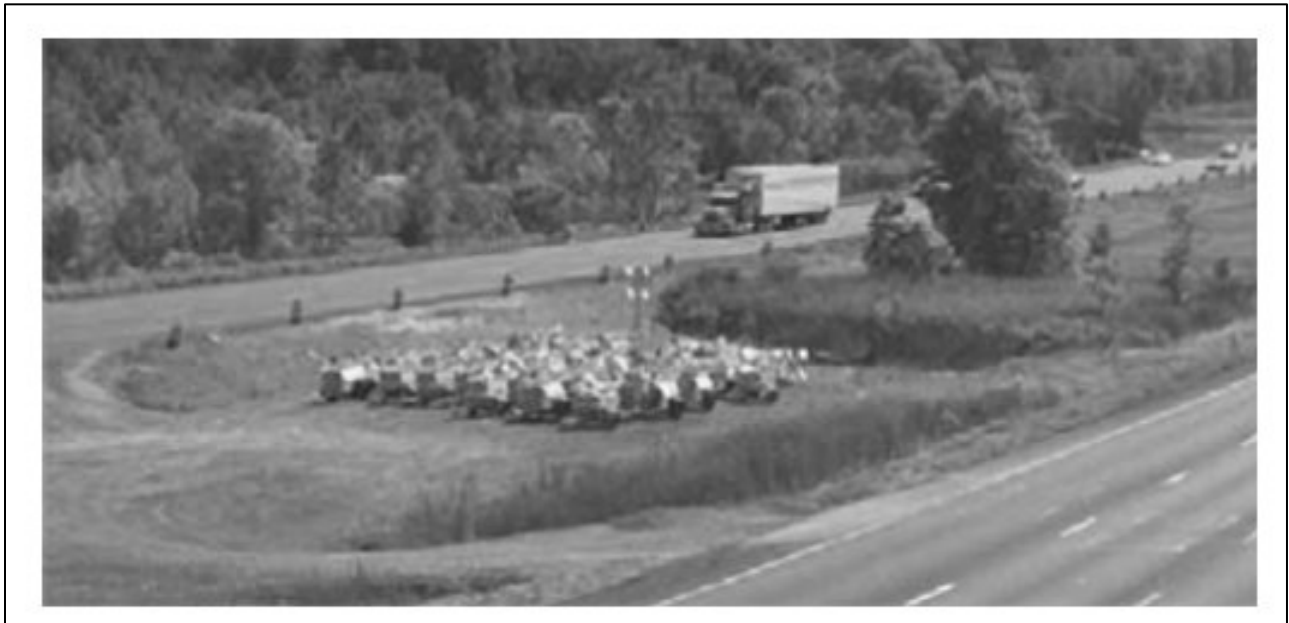
Figure 2.12: Equipment stored in median beyond roadside clear zone (Bryden and Mace, 2002)
