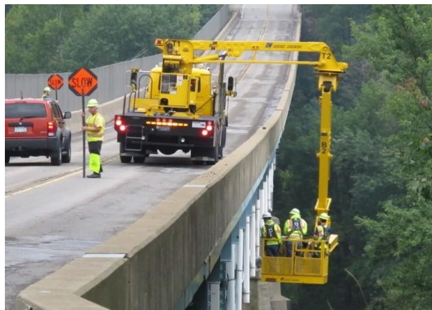
Figure 33 Bridge Manual Inspection through Crane (Source: Agile Assets)
