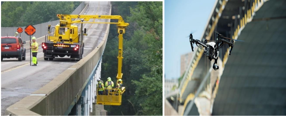
Figure 4.3 Bridge Visual Inspection through Crane and Drone (Source: Agile Assets)
