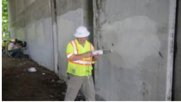
Figure 35 Bridge Non-Destructive Evaluation (NDE) (Source: Smart Sensys)
