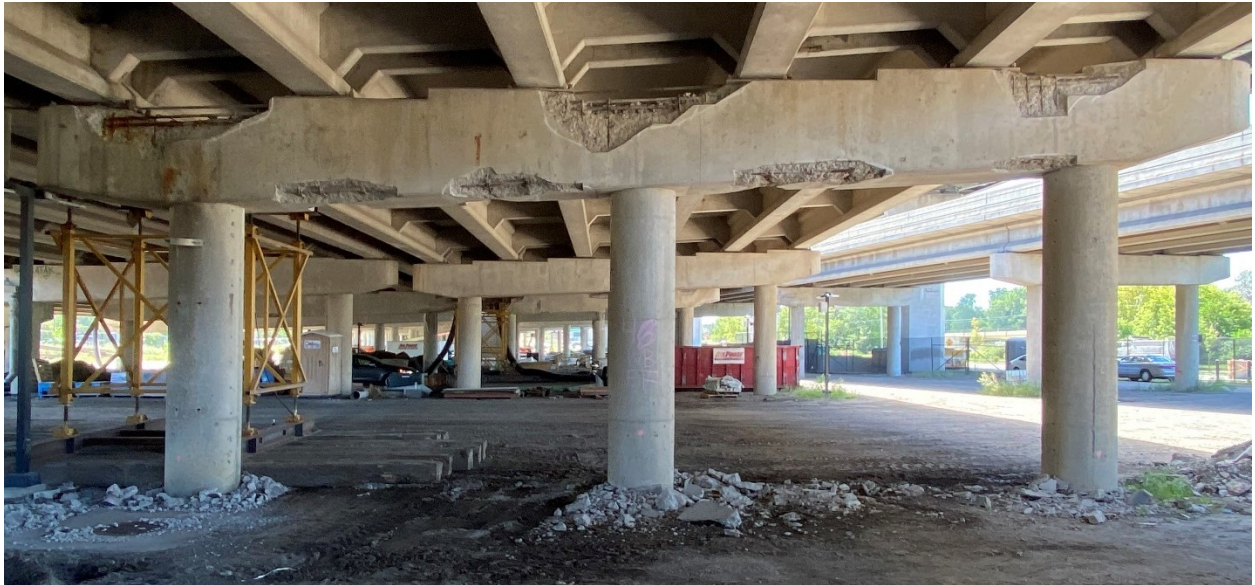
Figure A.36. East face of Pier 48EB
