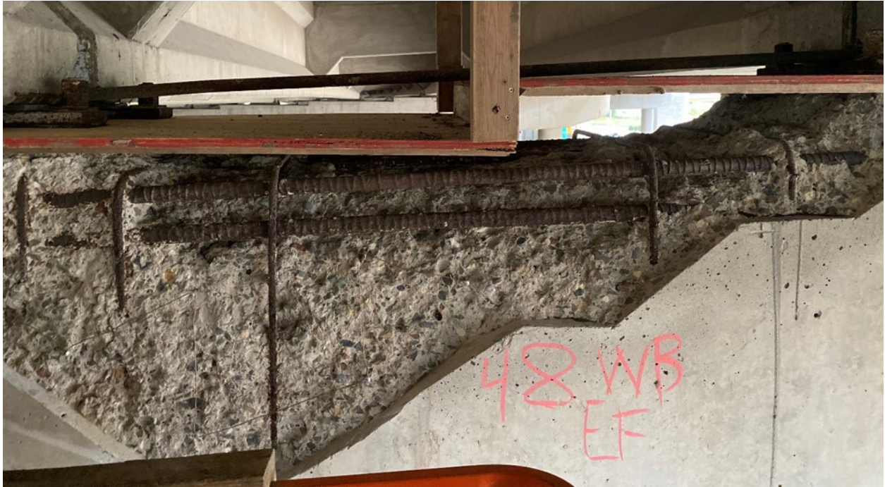
Figure A.41. East face of Pier 48EB
