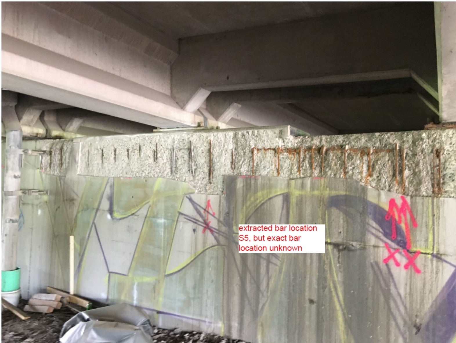
Figure B.9. Sample rebar collection sites during contract repairs
