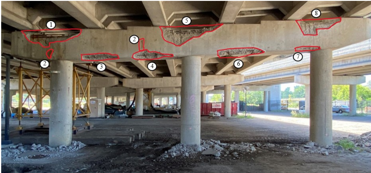
Figure 4.15. East face of Pier 48EB (photo taken in 2020)
