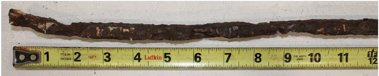
(h) S8 sample, #5 bar (50%-75% section loss)
