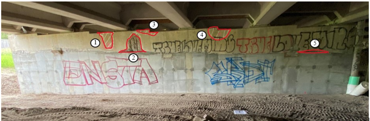
Figure 4.10. West face of Pier 21EB (photo taken in 2020)
