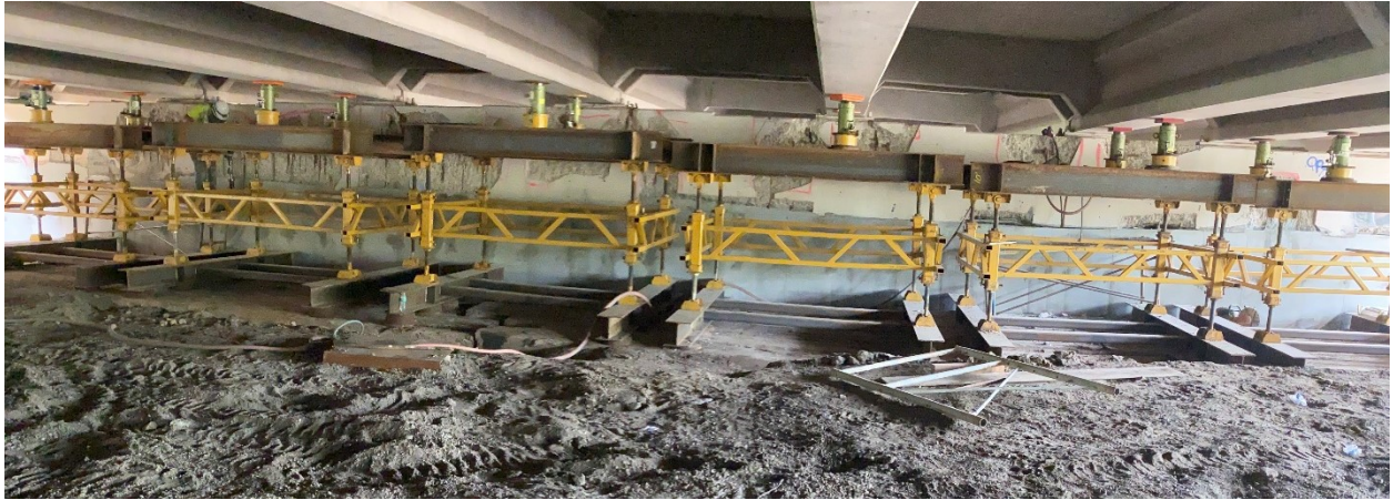
Figure A.1. East face of Pier 12WB
