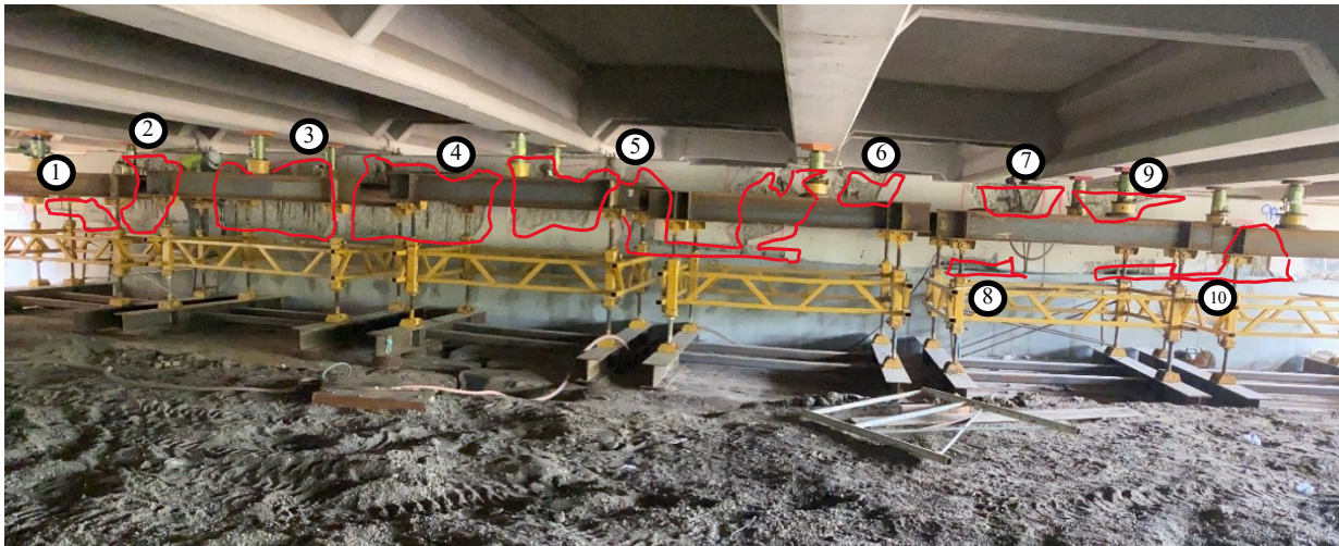
Figure 4.5. East face of Pier 12WB (photo taken in 2020)
