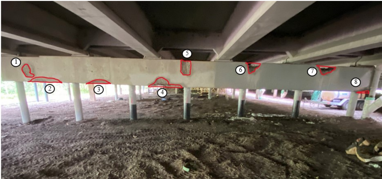
Figure 4.20. East face of Pier 15EB (photo taken in 2020)
