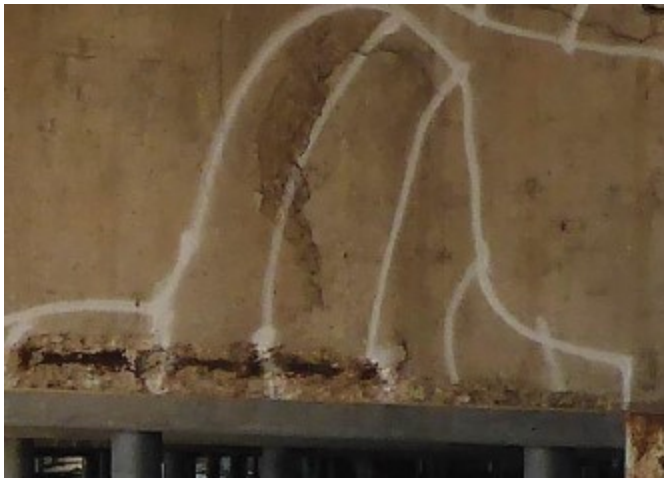
Figure 4.8. Location 7 of Pier 21EB
