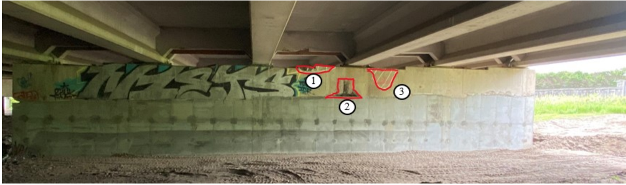
Figure 4.9. East face of Pier 21EB (photo taken in 2020)
