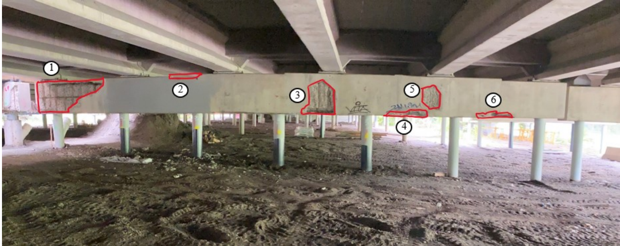
Figure 4.21. West face of Pier 15EB (photo taken in 2020)
