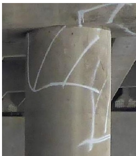
Figure 4.12. Location 9 of Pier 46WB
