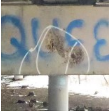
Figure 4.4. Location 14 of Pier 12WB
