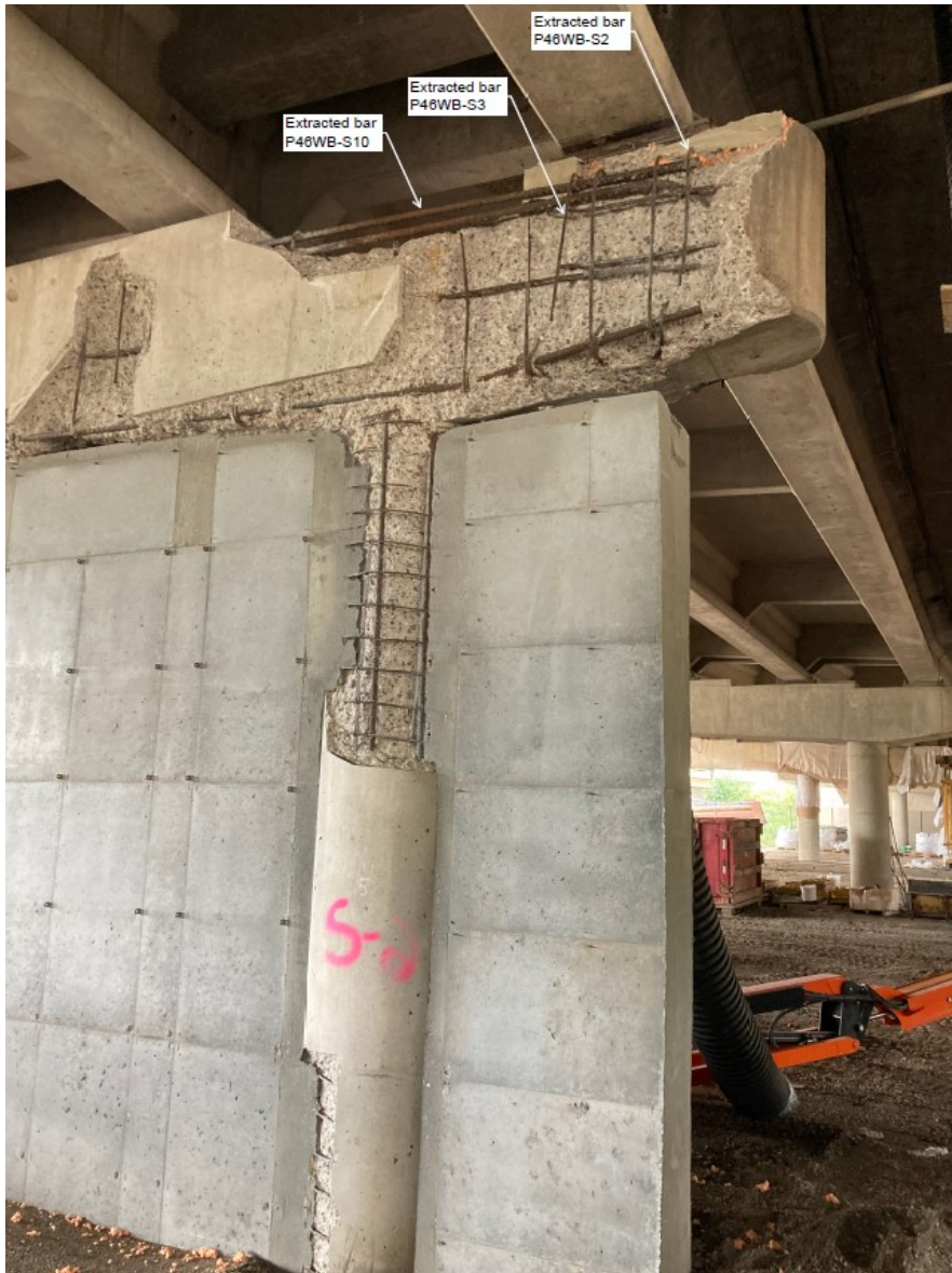
Figure B.6. Sample rebar collection sites during contract repairs
