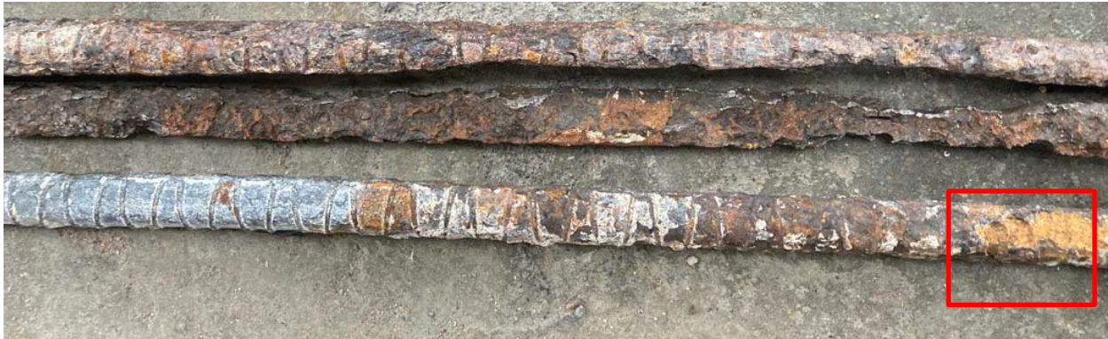
Figure 5.8. Rebar samples extracted from the bridge piers under consideration
