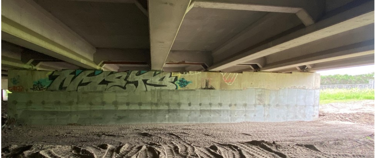
Figure A.29. West face of Pier 21EB
