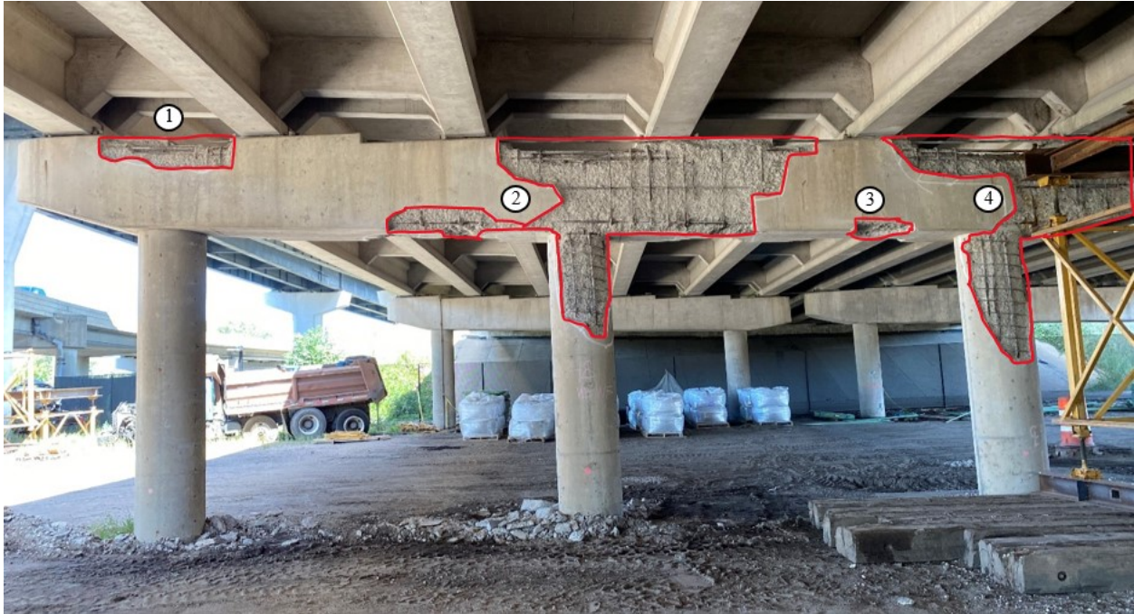
Figure 4.16. West face of Pier 48EB (photo taken in 2020)
