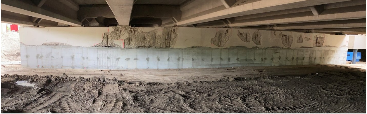
Figure A.5. West face of Pier 12WB
