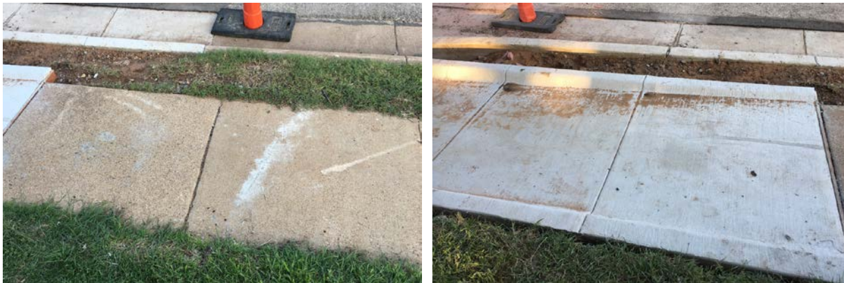
Figure 54. Pedestrian condition: old pedestrian (left) and recently constructed pedestrian (right)
