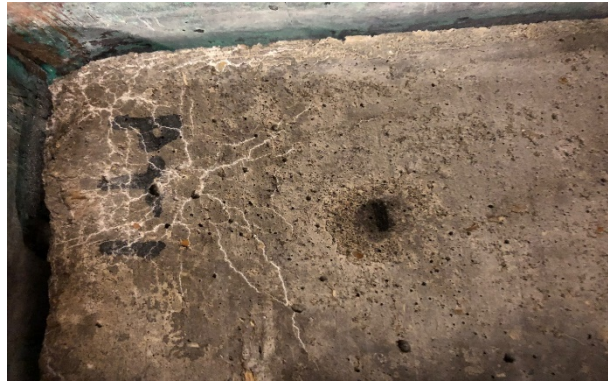
Figure 47. Surface of cycled prism concrete specimen, PT1
