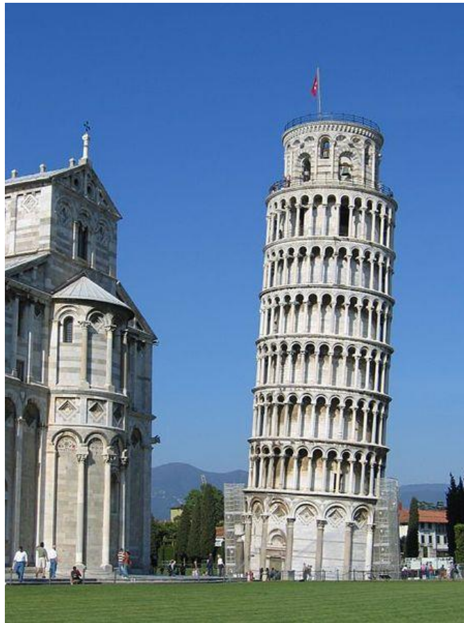
Figure 8. The Leaning Tower of Pisa (Retrieved from
