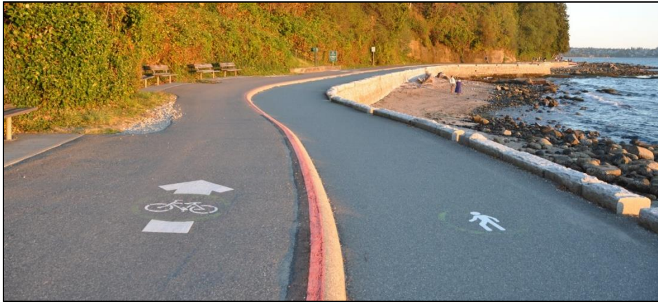
Figure 4: Paths in Stanley Park (Vancouver, British Columbia) include lane markings, separate paths, and one-way bicycle traffic to manage high active transportation volumes (photo by author).
