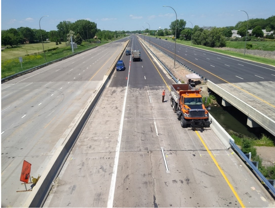
Figure F.12: Truck positioned at L1T4W of Bridge 27926.
