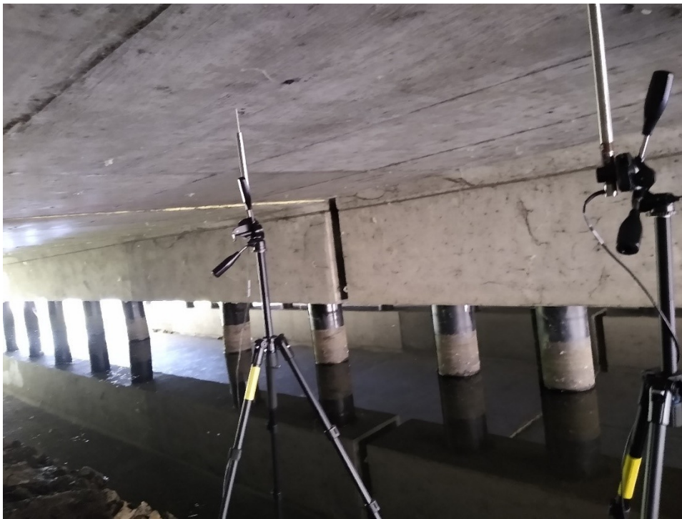
Figure F.6: LVDTs installed on the East span of Bridge 27926.
