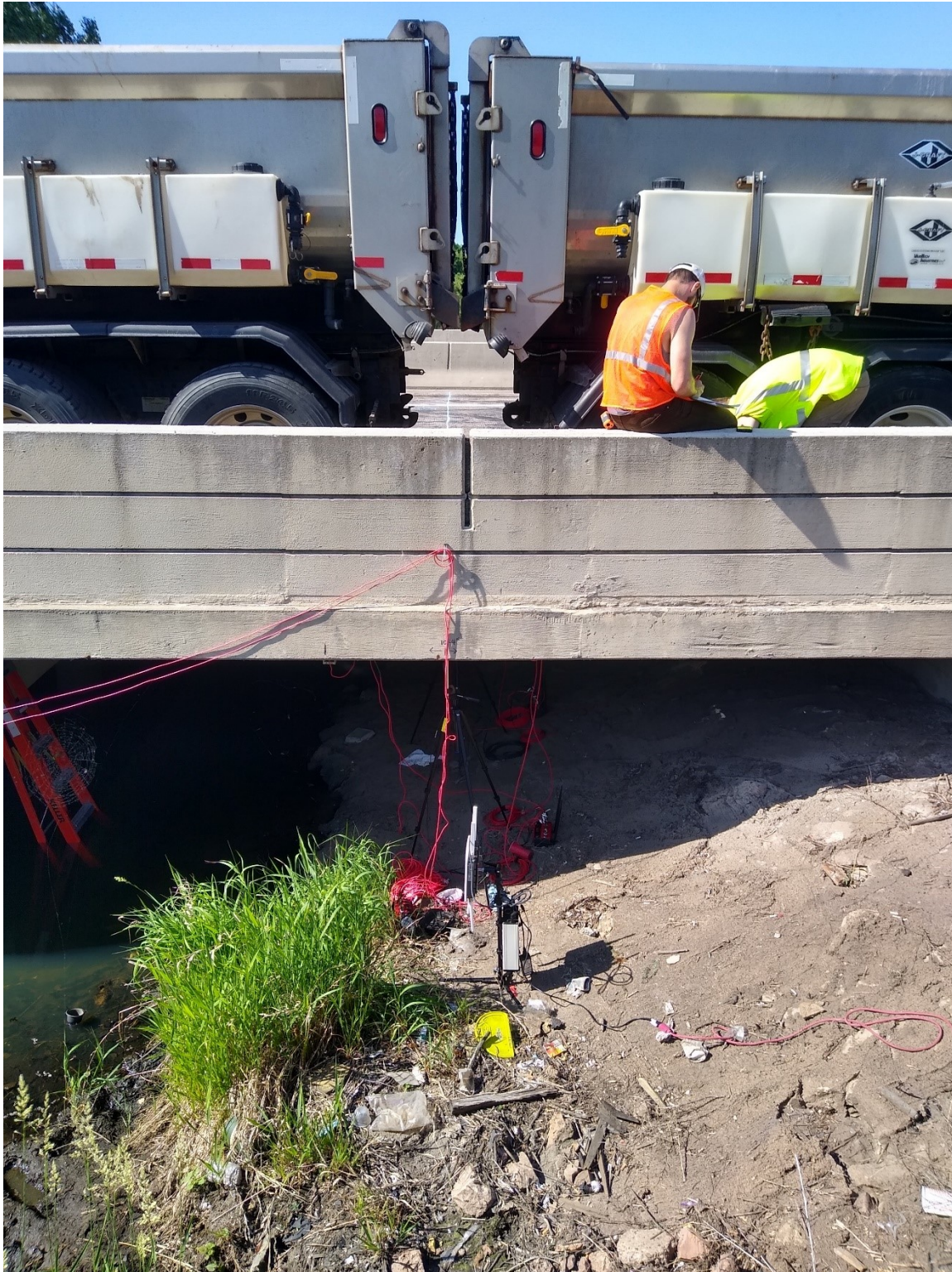
Figure F.11: Back-to-back truck tests on the West span of Bridge 27926 centered at midspan (deflection joint and instruments).
