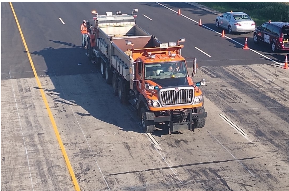
Figure H.10: Back-to-back trucks at West span of Bridge 27925 (L4T2W).
