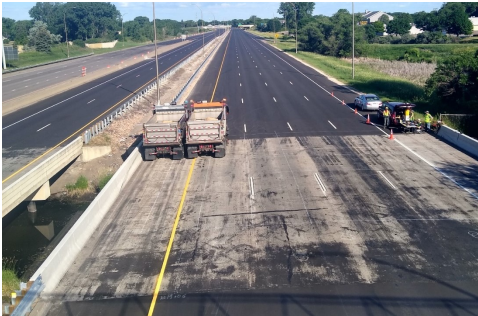
Figure H.14: Side-by-side trucks at West span of Bridge 27925.
