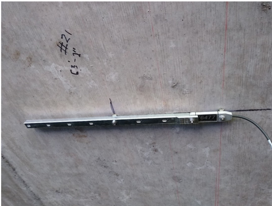
Figure H.2: Strain gauge installed on the West span of Bridge 27925.
