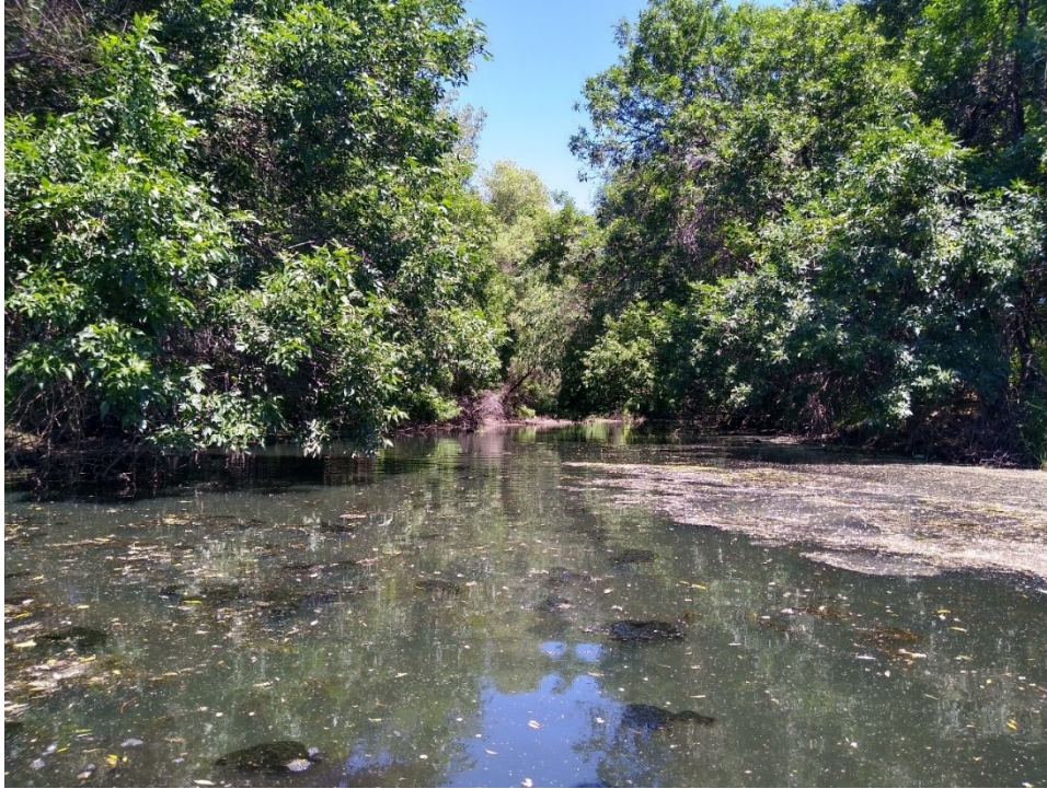
Figure H.3: View North from midspan of Bridge 27925.
