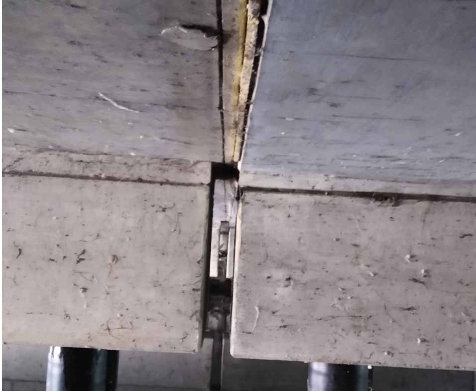
Figure A.11: Expansion joint between Bridge 27909 and Bridge 27926.
