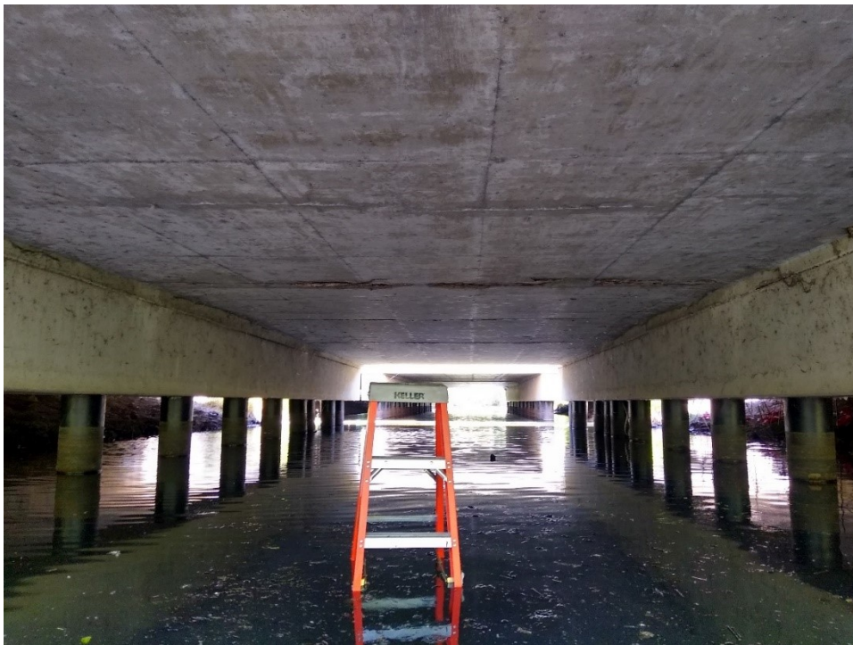
Figure H.4: Center span of Bridge 27925 before installation of accelerometers.
