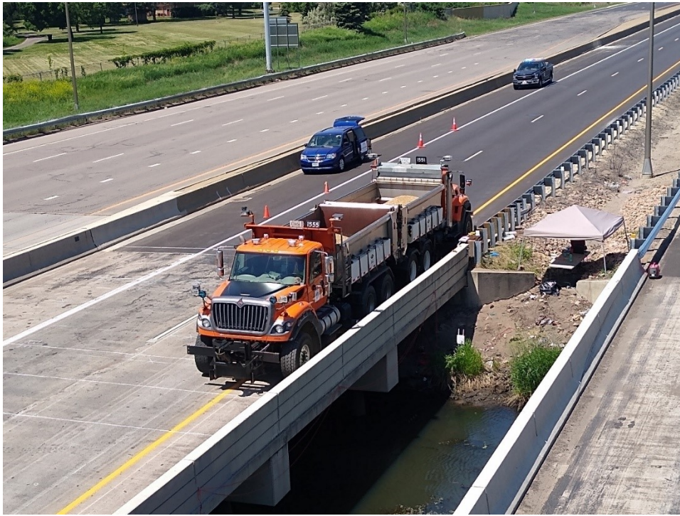
Figure F.15: Back-to-back trucks at West span of Bridge 27926.
