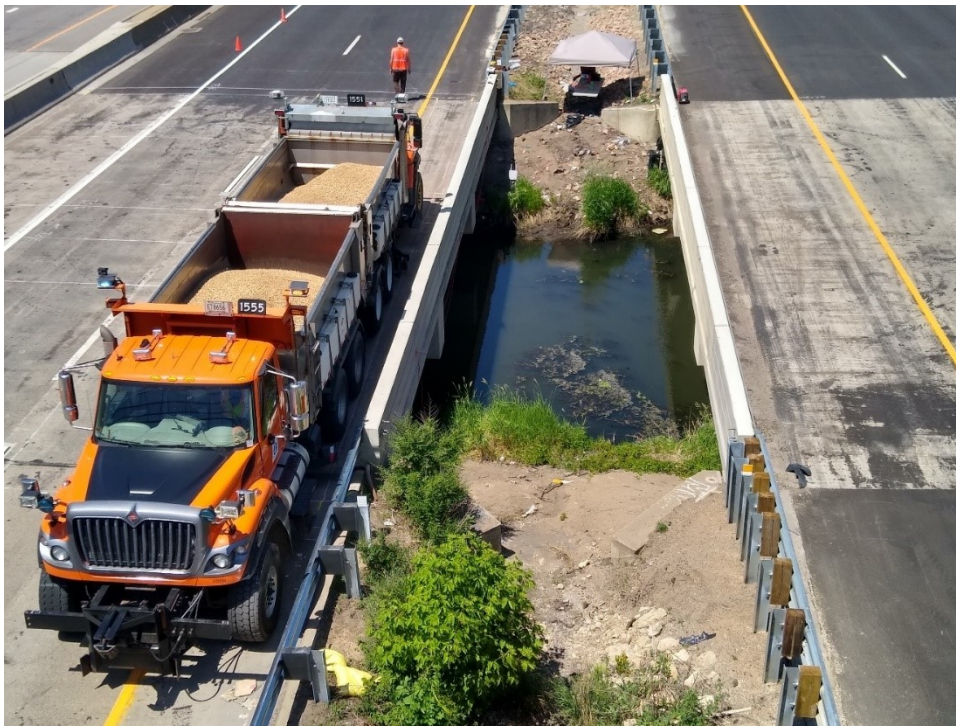
Figure F.17: Back-to-back trucks at East span of Bridge 27296.
