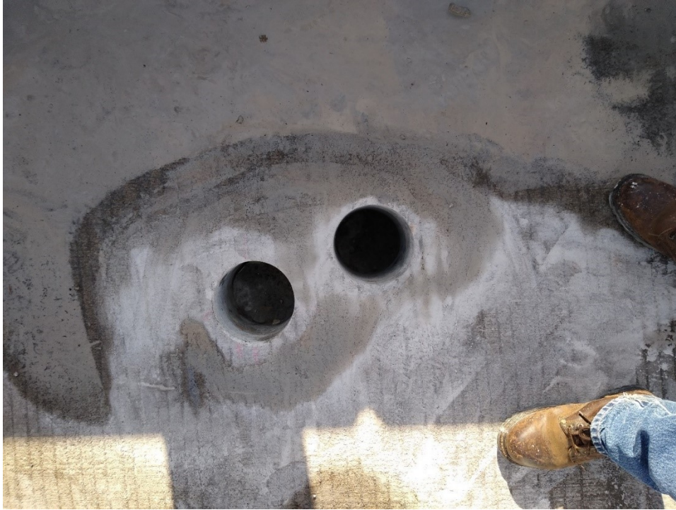
Figure B.5: 6 in. cored holes in Bridge 27926.
