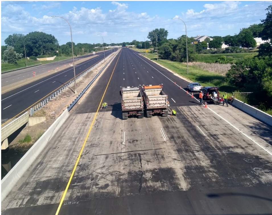
Figure H.16: Side-by-side trucks at West span of Bridge 27925.
