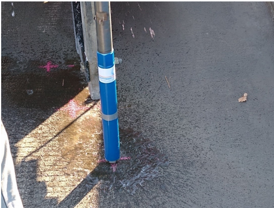
Figure B.2: Drilling 1.75 in. cores from Bridge 27926.
