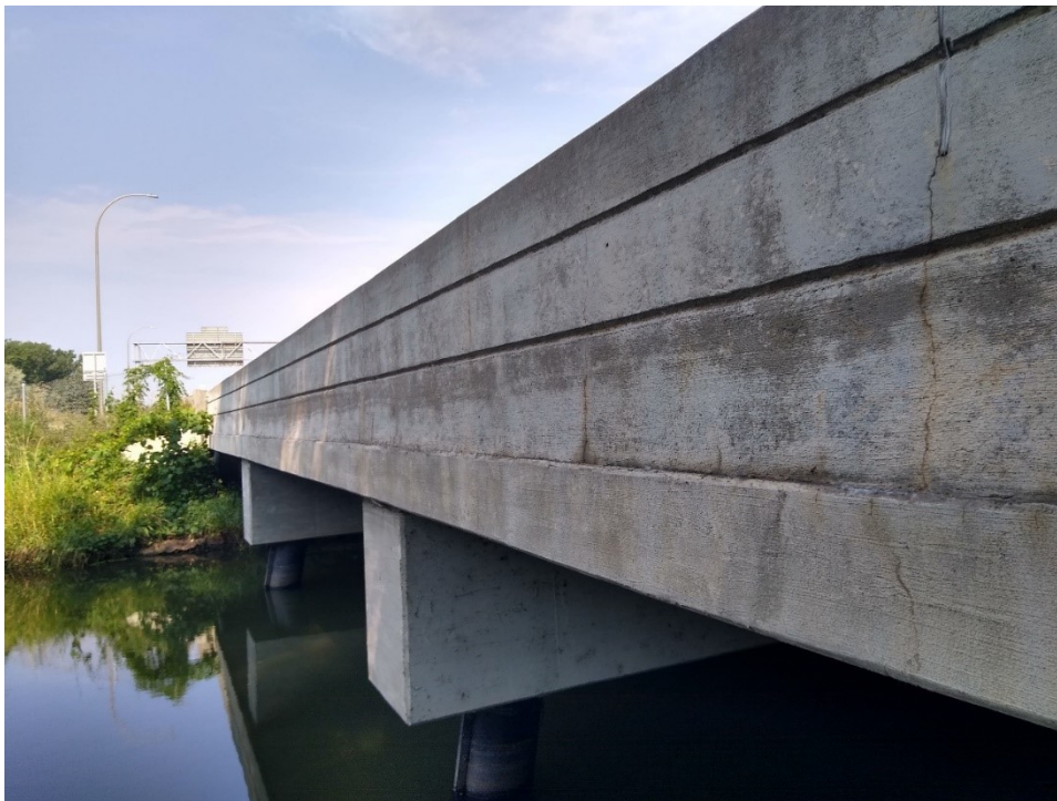
Figure A.4: North edge of Bridge 27909.
