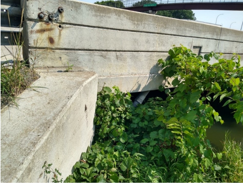
Figure A.9: Abutment and barrier of Bridge 27909 from the South.
