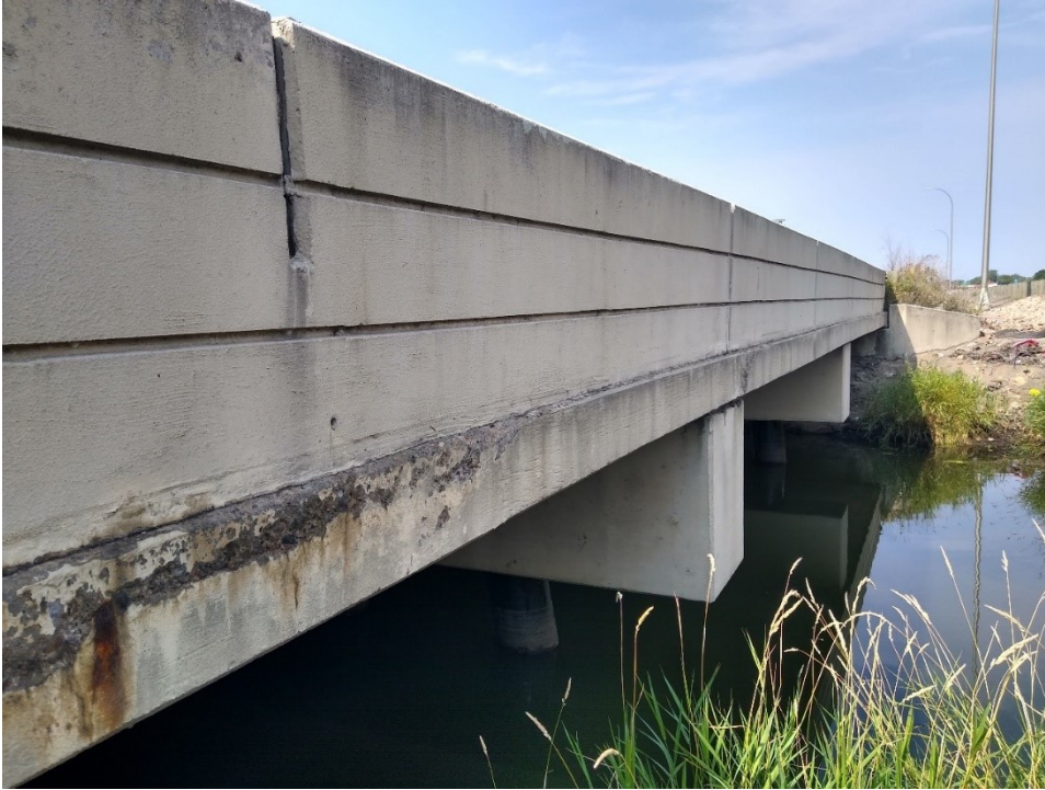
Figure A.5: South edge of Bridge 27926 (Primary testing structure).
