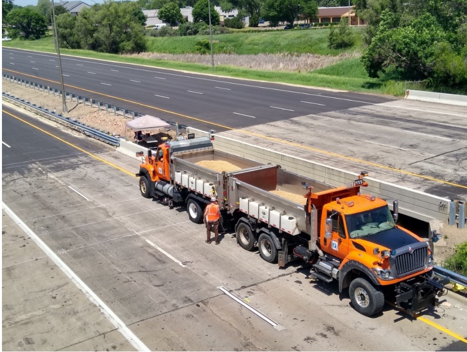
Figure F.16: Back-to-back trucks at East span of Bridge 27926.
