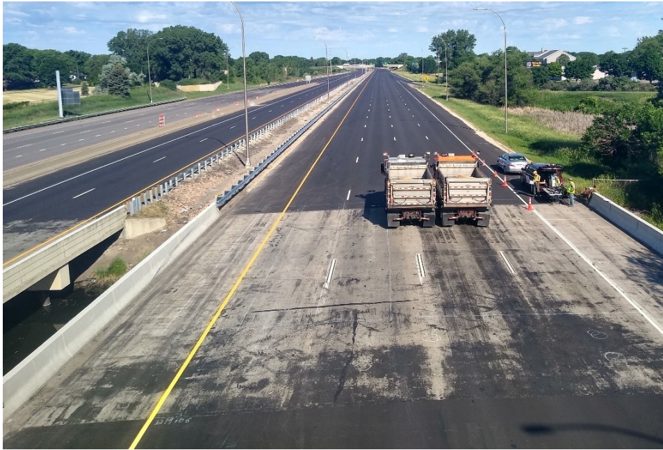
Figure H.17: Side-by-side trucks at West span of Bridge 27925.
