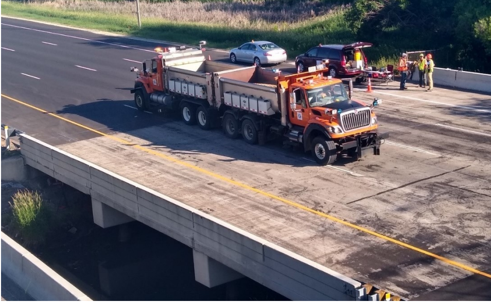
Figure H.11: Back-to-back trucks at West span of Bridge 27925 (L4T1W).
