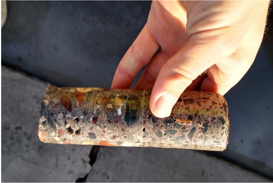
Figure B.3: 1.75 in. core from Bridge 27926.
