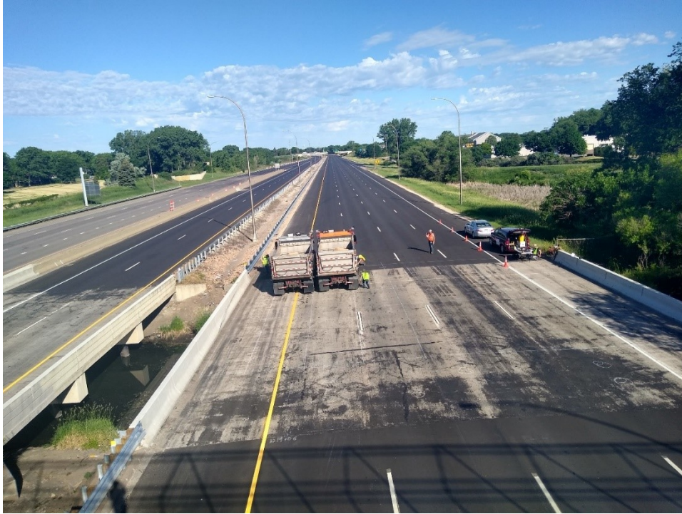
Figure H.15: Side-by-side trucks at West span of Bridge 27925.
