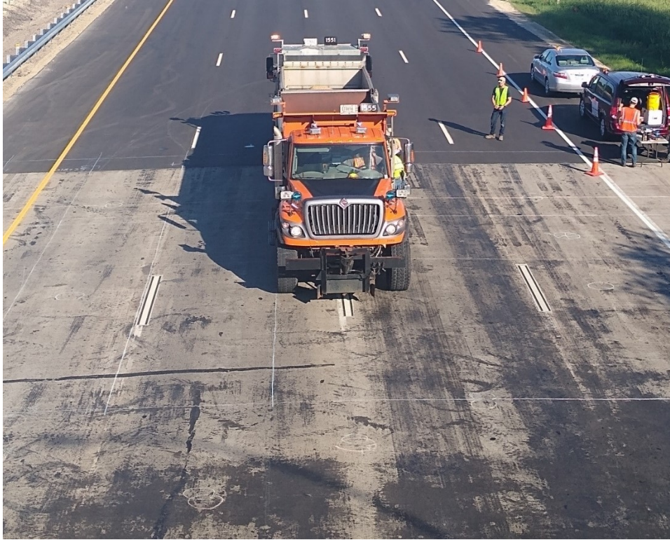
Figure H.13: Back-to-back trucks at West span of Bridge 27925 (L5T1W).
