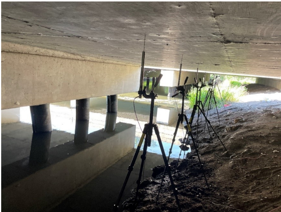
Figure 3.16: LVDTs set up under Bridge 27926 during live load testing.
