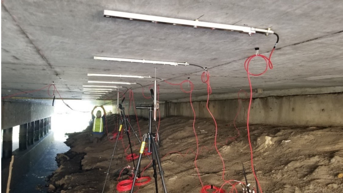
Figure 3.17: Strain gauges installed under Bridge 27926 during live load testing.
