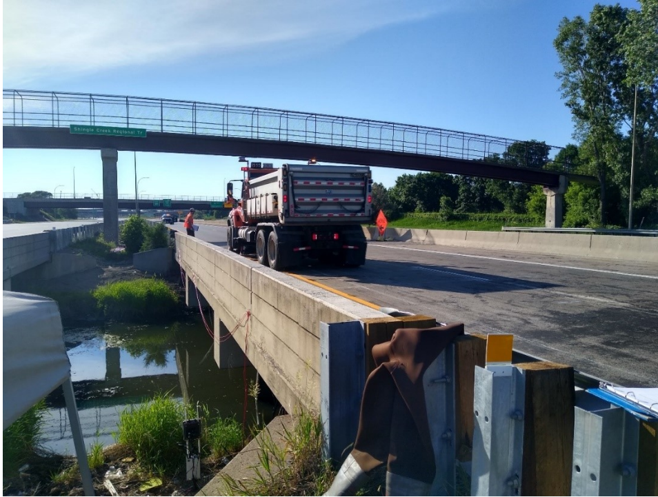
Figure F.7: Truck positioned at L2T4W (4.5 ft from the barrier and midspan of center span) on Bridge 27926 during live load testing.
