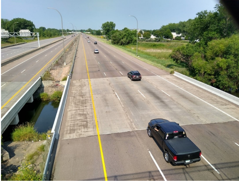
Figure A.3: Bridge 27925 from the East.
