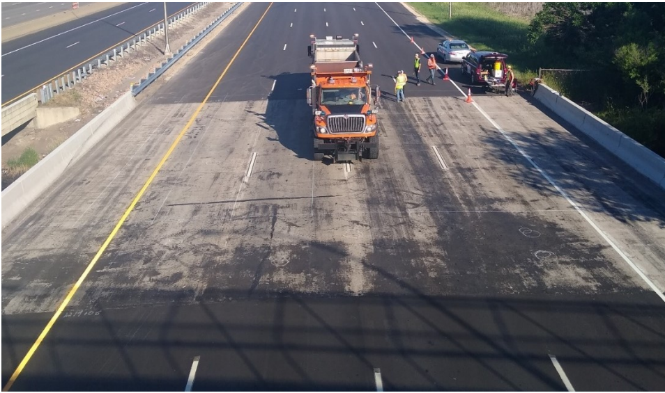
Figure H.12: Back-to-back trucks at West span of Bridge 27925 (L5T1W).
