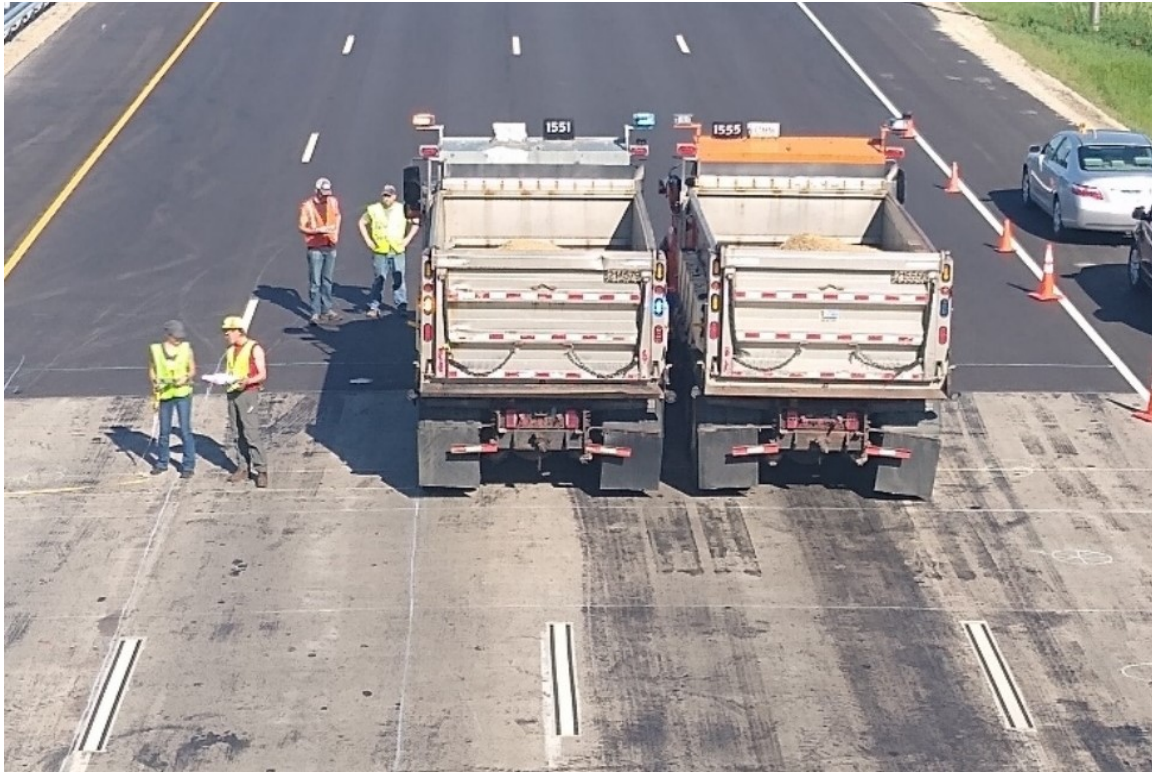
Figure 3.21: Side-by-side truck test.
