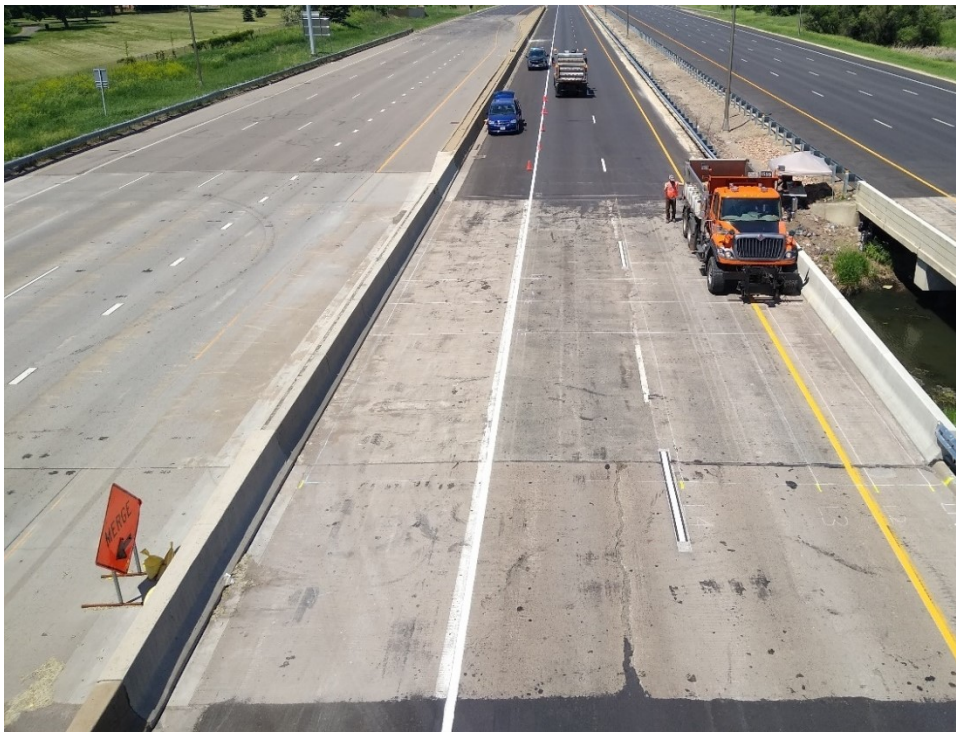
Figure F.13: Truck positioned at L1T2W of Bridge 27926.
