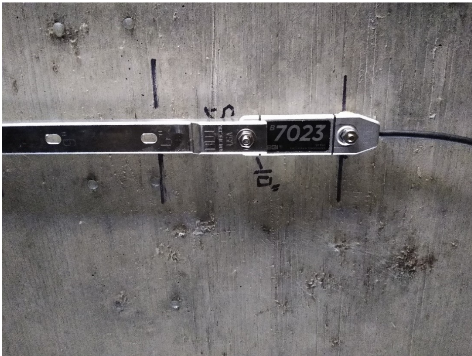
Figure F.4: Bridge Diagnostics strain gauge.
