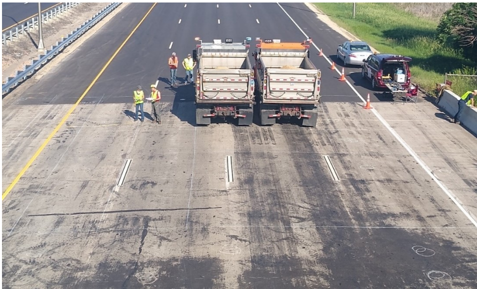
Figure H.18: Side-by-side trucks at West span of Bridge 27925.
