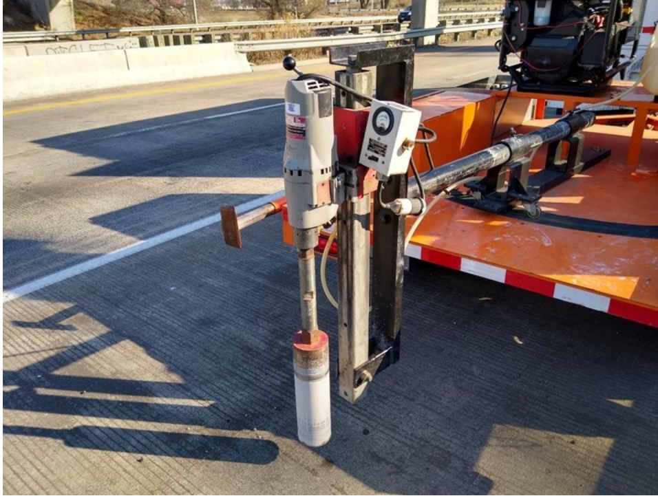
Figure B.1: MnDOT drill rig used for bridge deck coring.
