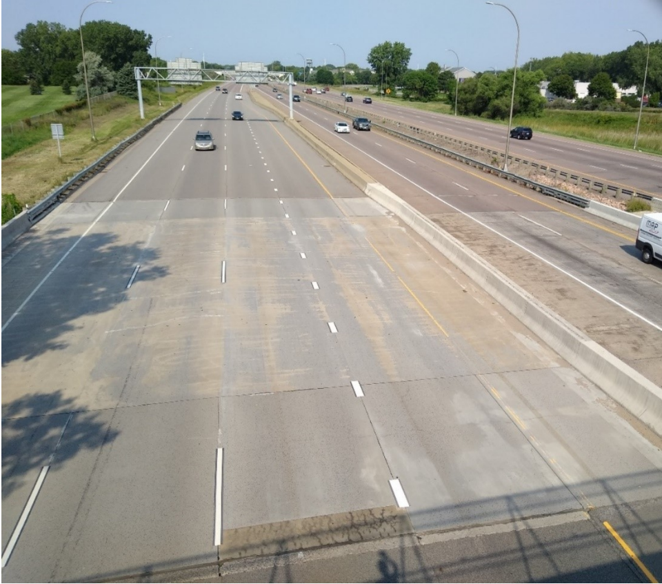
Figure A.1: Bridge 27909 from the East.
