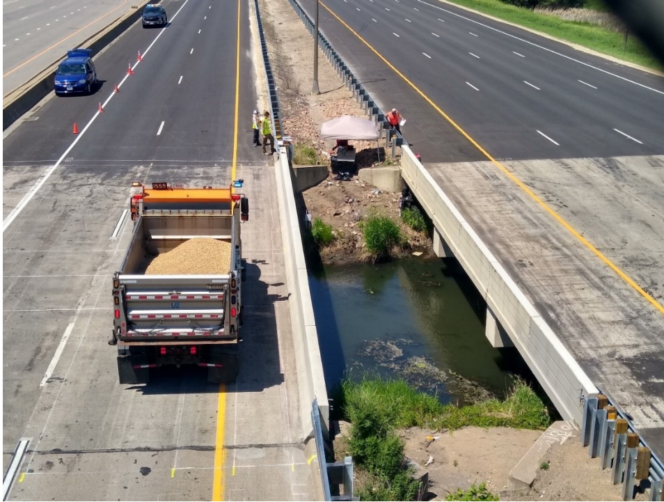
Figure F.18: Single truck at L2T1E on Bridge 27926.
