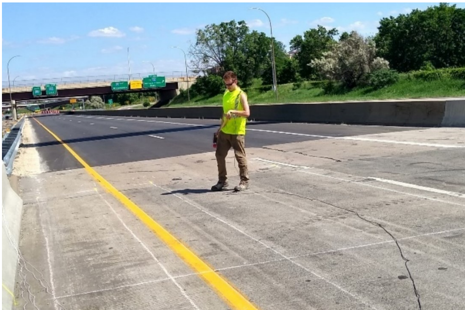
Figure F.19: Dynamic impact hammer testing on Bridge 27926.
