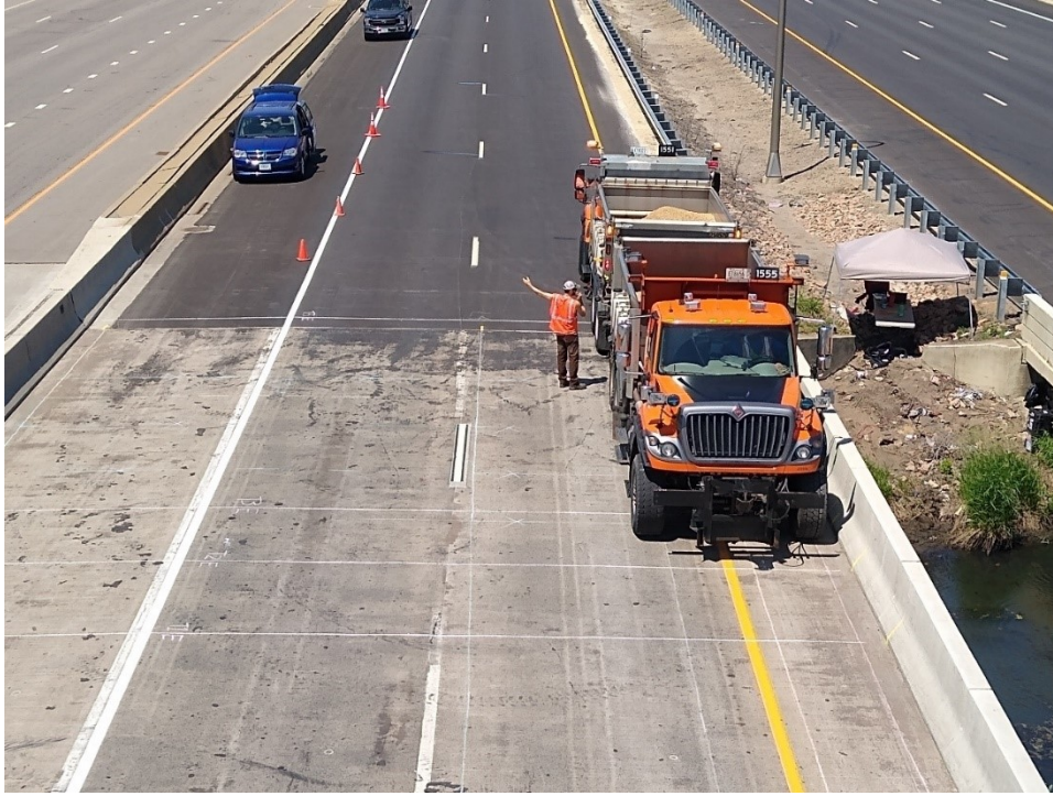
Figure F.14: Back-to-back trucks at West span of Bridge 27926.
