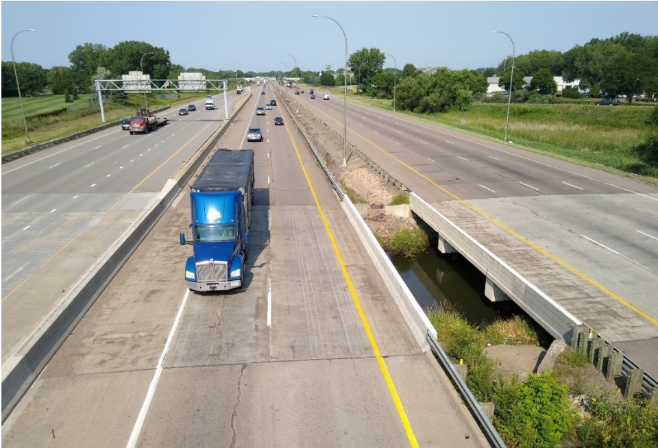
Figure A.2: Bridge 27926 from the East.
