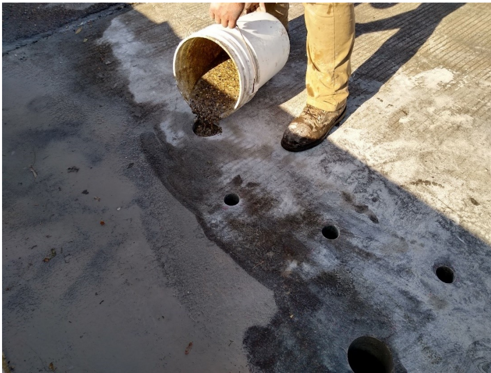
Figure B.6: Aggregate-epoxy resin fill.
