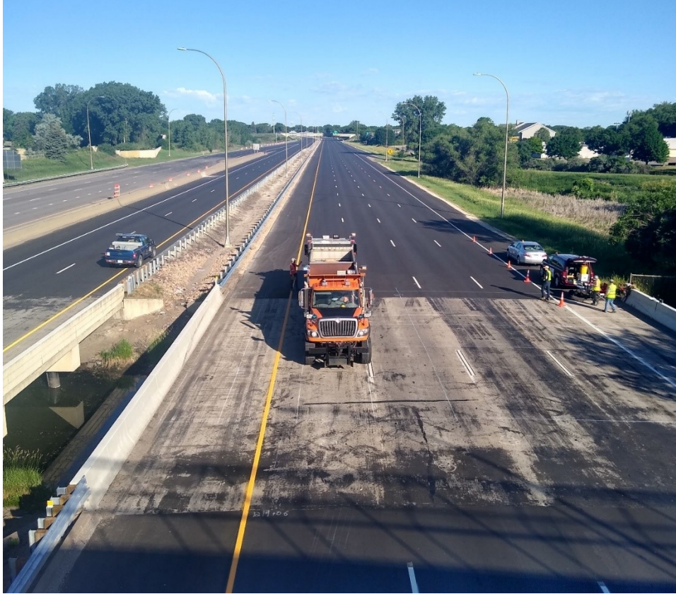
Figure H.9: Back-to-back trucks at West span of Bridge 27925 (L3T1W).
