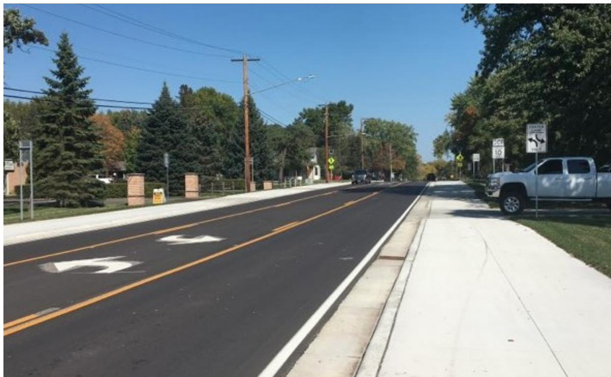
Figure 3.27 Watertown Highway 25, post-reconstruction
