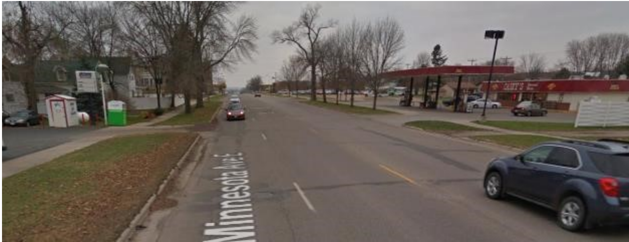
Panel A: Highway 28/Minnesota Avenue prior to the construction (2015)
