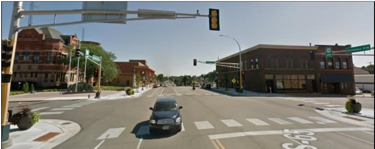
Panel B: Highway 95/ South Broadway Avenue after the reconstruction project (2016)
