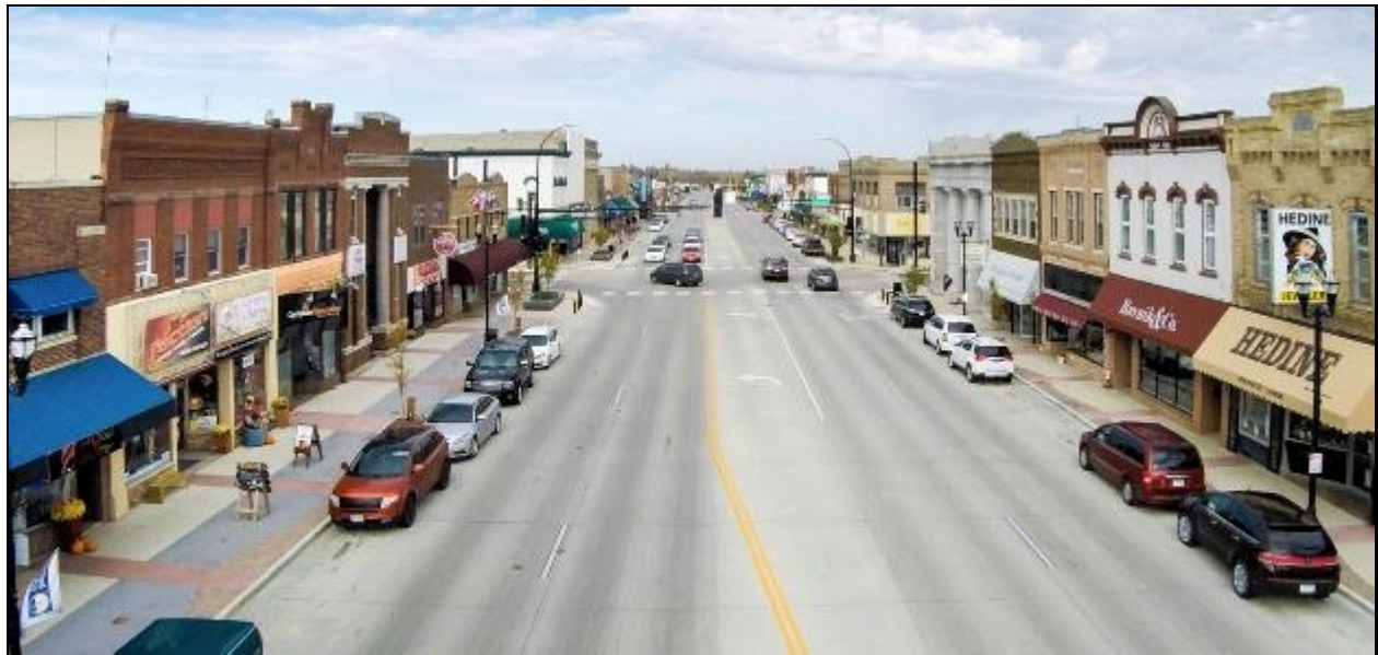
Figure 3.10 Alexandria Highway 65/South Broadway Avenue, post-reconstruction
