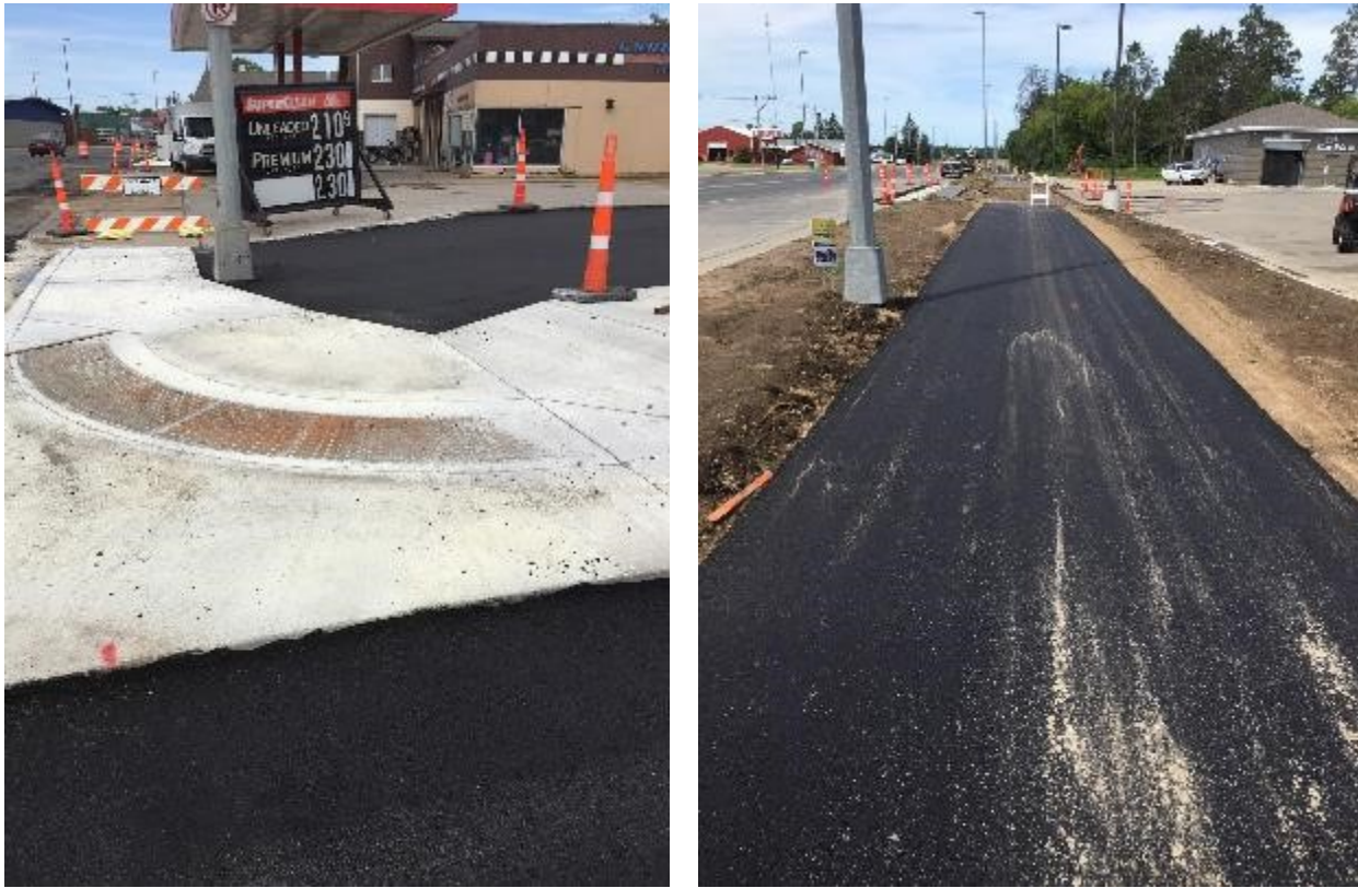
Figure 3.12 Installation of Bagley multi-use trail
