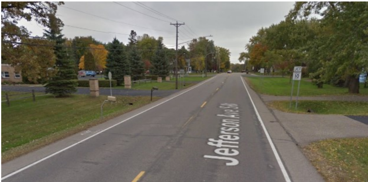
Figure 3.26 Watertown Highway 25, pre-reconstruction
