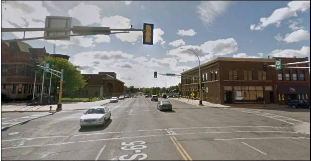
Panel A: Highway 95/ South Broadway Avenue before the reconstruction project (2013)
