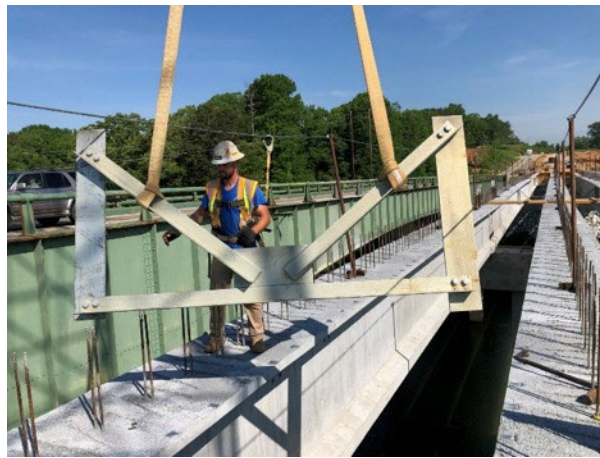
Figure 11. Photo. Installation of k-frame diaphragm
