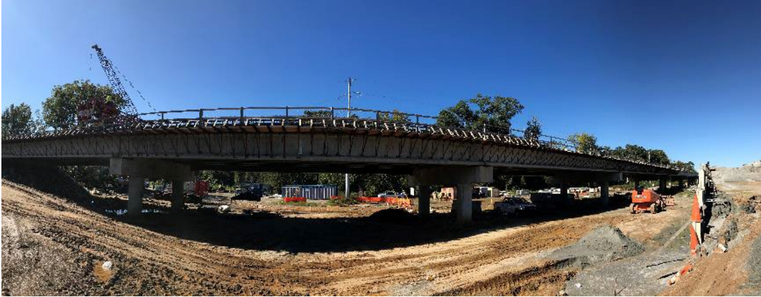
Figure 43. Photo. Panoramic picture of Span27RT
