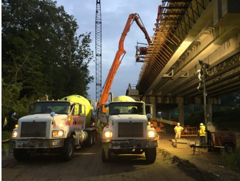
Figure 60. Photo. Deck pour on August 26, 2020
