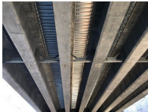
Figure 2. Photo. Intermediate k-frame diaphragms in situ
