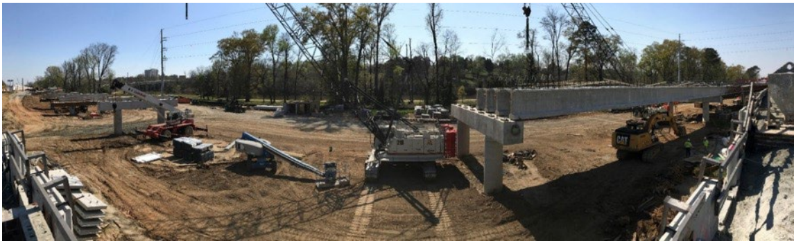
Figure 48. Photo. End of span prior to concrete deck pour
