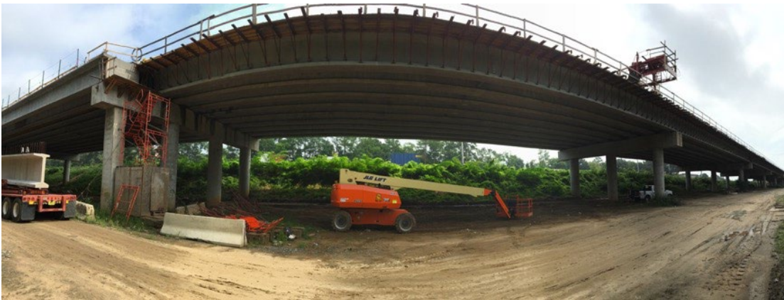
Figure 49. Photo. Panoramic photo of span prior to deck pour
