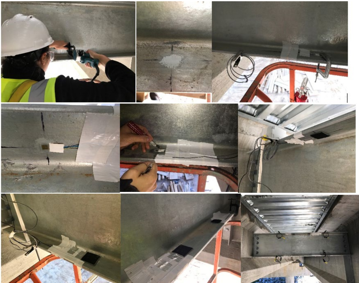
Figure 45. Photo. Collection of pictures depicting strain gauge installation process
