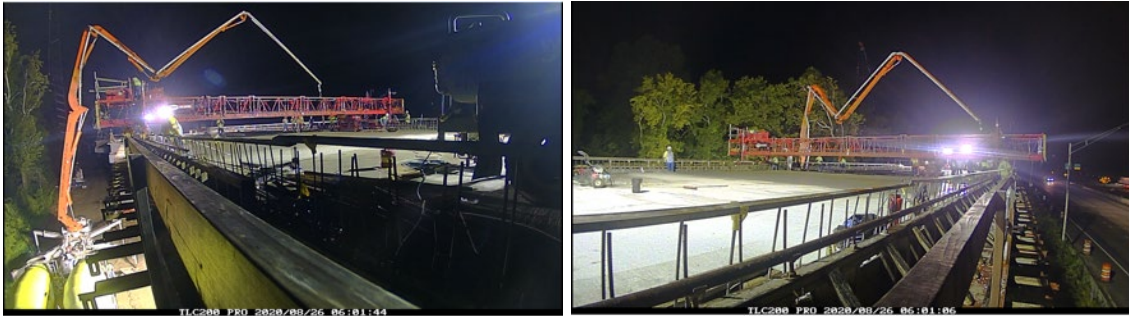
Figure 62. Photo. Time-lapse camera footage on both sides of the bridge
