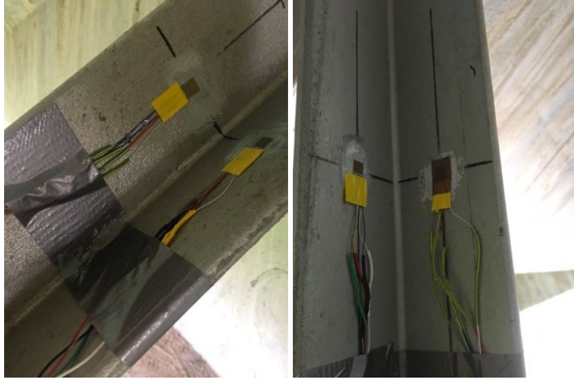
Figure 57. Photo. Strain gauges after bonding to surface
