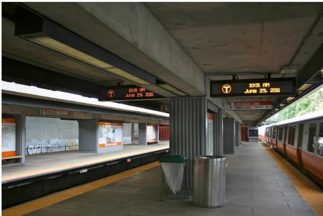
Figure 2.4: Sullivan Square, Southbound Orange Line Platform
