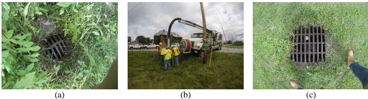
Figure B.12: VJT Operations Using Vactor 2100 on June 27, 2018 in Union County (a) Structure prior to cleaning, (b) Cleaning of Structure, (c) Structure post cleaning.
