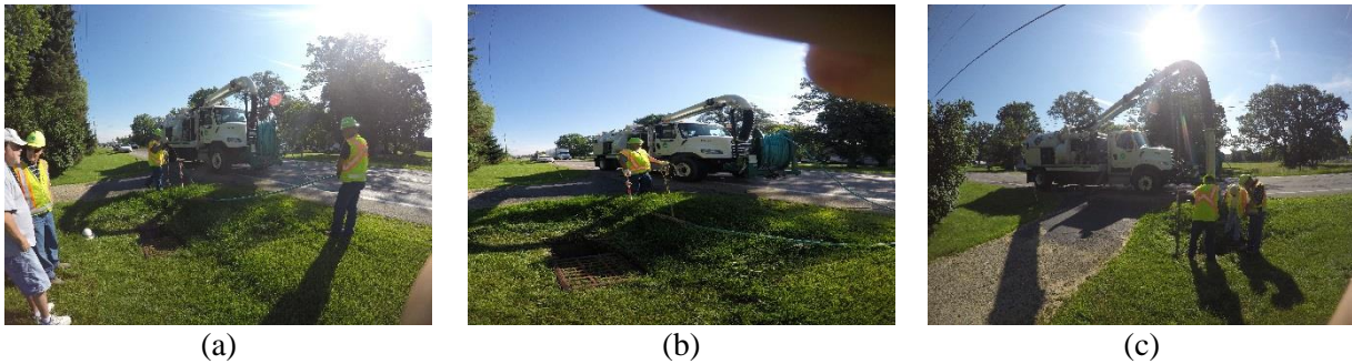
Figure B.6: VJT Operations Using Vac-Con 9CY on June 26, 2018 in Madison County (a, b) Work setup, (c) Cleaning of the structure.
