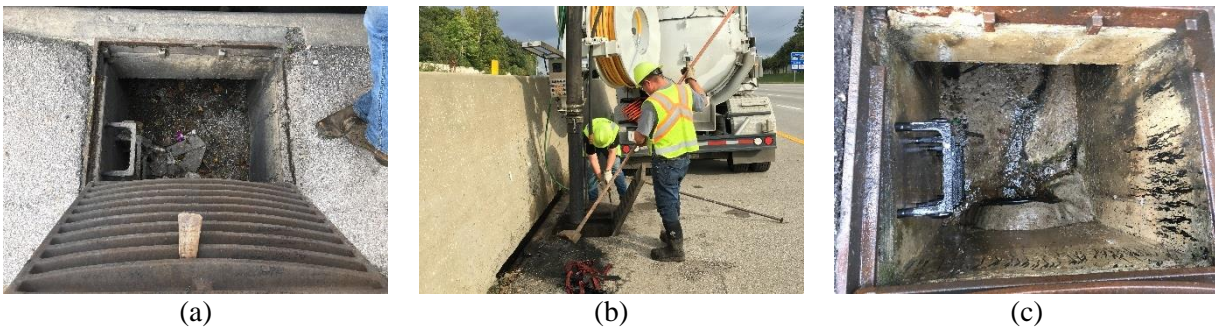
Figure B.58: BUCHER RECYcler 315 Operations on October 4, 2018 in Franklin County (a) Structure prior to cleaning, (b) During cleaning, (c) Structure after the cleaning processes.
