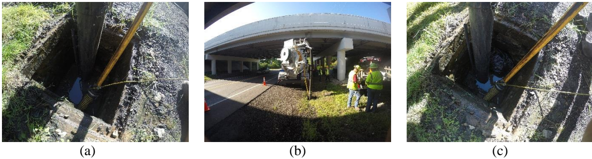
Figure B.26: BUCHER RECycler 315 Training Operations on July 11, 2018 (a) Simultaneous cleaning and jetting of structure, (b) Equipment zone, (c) Large debris within structure.
