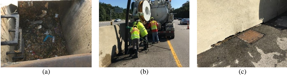
Figure B.65: BUCHER RECyler Operations on October 9, 2018 in Franklin County (a) Structure prior to cleaning, (b, c) Operators running vacuum and jet on structure and after cleaning.
