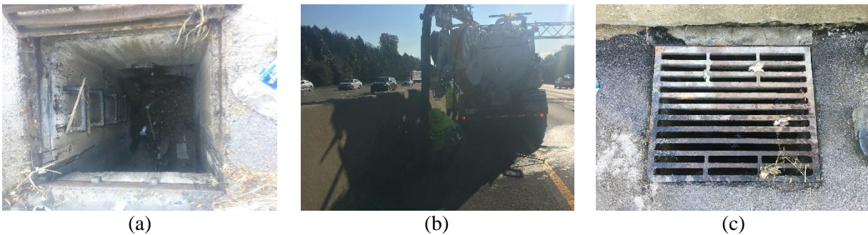
Figure B.59: BUCHER RECYcler Operations on October 9, 2018 in Franklin County (a) Structure prior to cleaning, (b) Cleaning operations, (c) Structure after cleaning.
