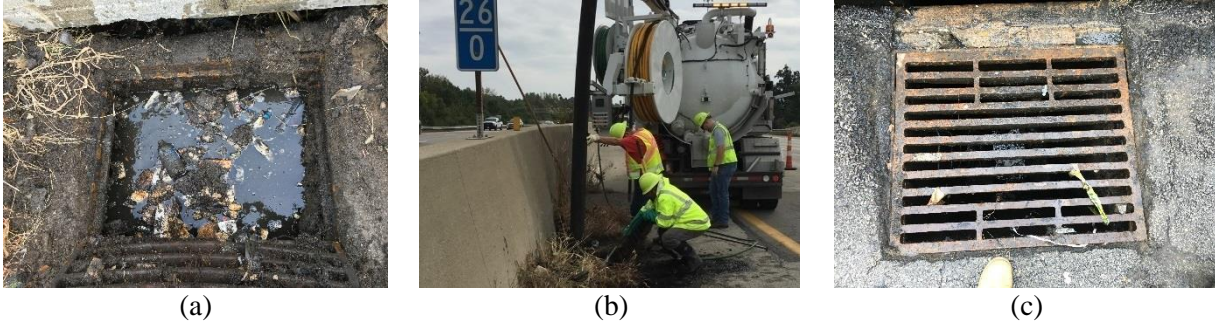
Figure B.53: BUCHER RECycler 315 Operations on October 2, 2018 in Franklin County (a) Structure prior to cleaning, (b) operators clearing in and around catch basin, (c) post cleaning.
