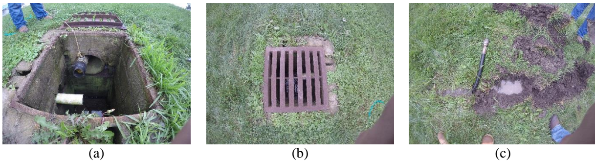
Figure B.11: VJT Operations Using Vactor 2100 on June 27, 2018 in Union County (a) Structure prior to cleaning, (b) Structure post cleaning, (c) Searching for collapsed pipe.
