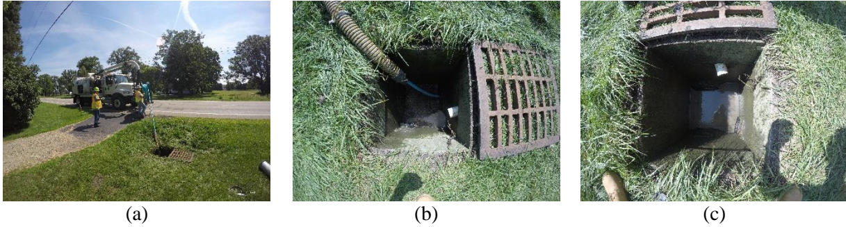
Figure B.5: VJT Operations Using Vac-Con 9CY on June 26, 2018 in Madison County (a) Work setup, (b) Cleaning of the structure, (c) Structure post cleaning.
