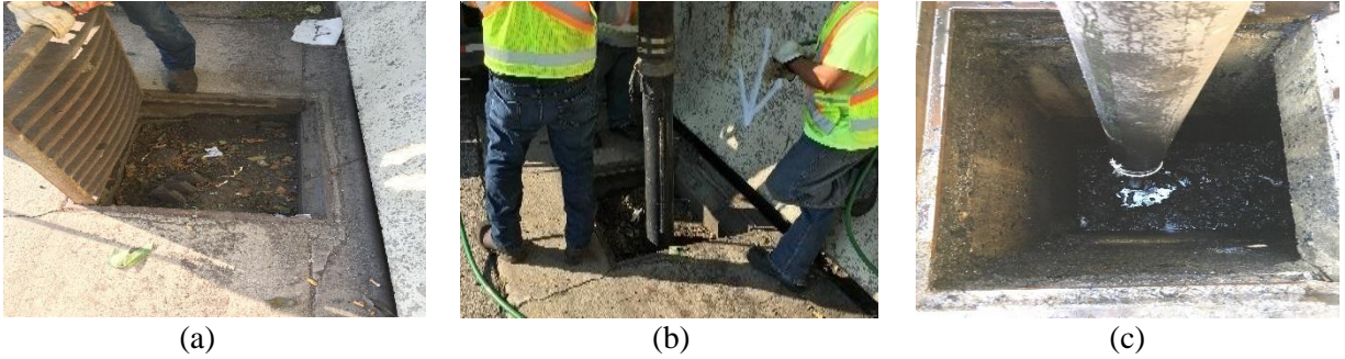
Figure B.45: BUCHER RECycler 315 Operations on August 28, 2018 in Franklin County (a) Structure prior to cleaning, (b) Cleaning of the structure, (c) Structure post cleaning.
