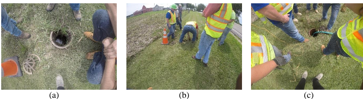
Figure B.4: VJT Operations Using Vac-Con 9CY on June 25, 2018 in Franklin County (a) Structure prior to cleaning, (b) Cleaning of the structure, (c) Jetting through structure line.
