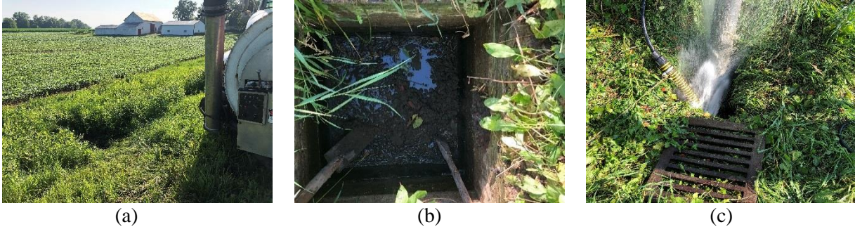
Figure B.15: VJT Operations Using Vactor 2100 on June 28, 2018 in Union County (a) Zone prior to cleaning, (b) Inner structure prior to cleaning, (c) Cleaning of the structure.
