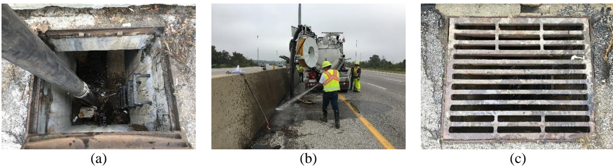
Figure B.56: BUCHER RECycler 315 Operations on October 3, 2018 in Franklin County (a) Vacuum operating on structure, (b) Cleaning debris around cavity, (c) Structure post cleaning.
