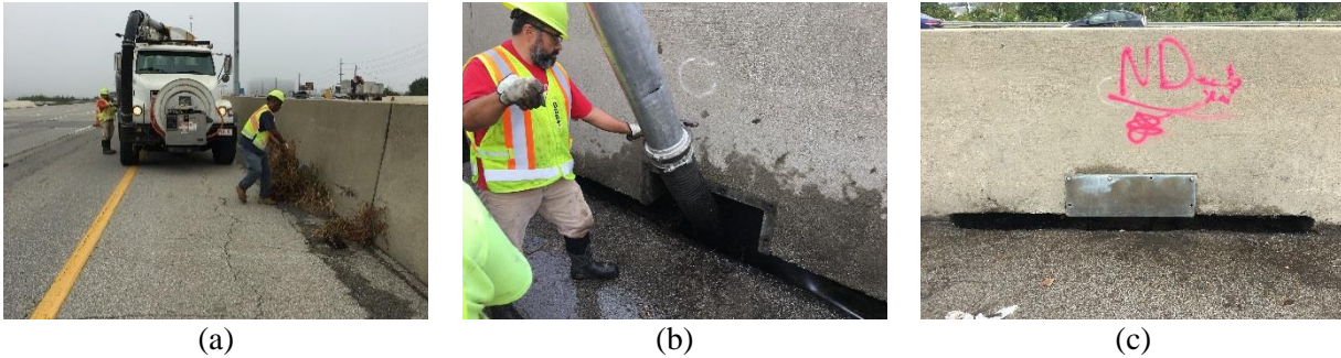
Figure B.57: Vactor 2100 Operations on October 3, 2018 in Franklin County (a) Operators setting up zone, (b) Performing vacuum on structure, (c) Gutter after cleaning.
