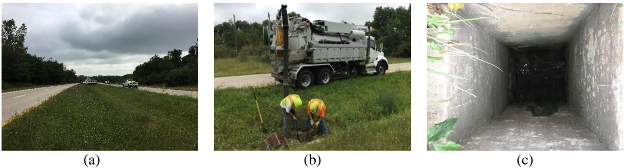
Figure B.47: BUCHER RECycler 315 Operations on August 30, 2018 in Madison County (a) Operators setting up zone, (b) Cleaning of the structure, (c) Structure post cleaning.
