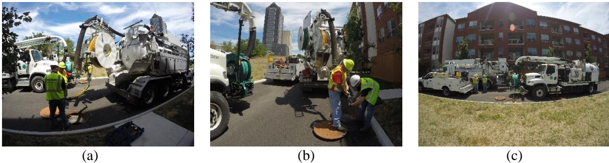
Figure B.42: BUCHER RECYcler 315 Operations on July 19, 2018 in Franklin County (a) The RECYcler and Vac-Con preparing, (b) RECYcler running the jet, (c) Vac-Con jetting structure.
