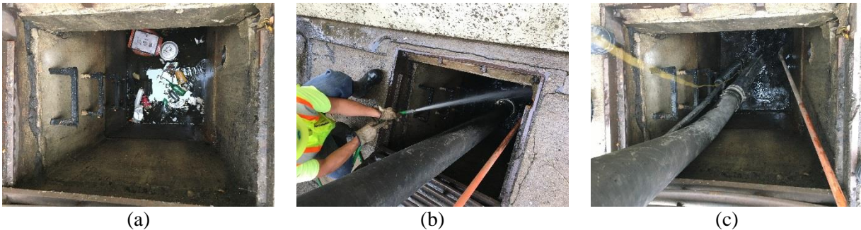
Figure B.50: BUCHER RECycler 315 Operations on September 26, 2018 in Franklin County (a) Structure prior to cleaning, (b) Cleaning of the structure, (c) Structure post cleaning.
