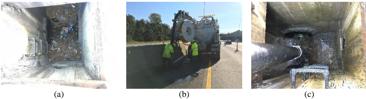
Figure B.60: BUCHER RECYcler Operations on October 9, 2018 in Franklin County (a) Structure prior to cleaning, (b, c) During cleaning operations.
