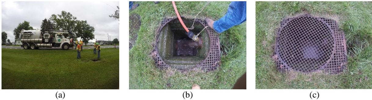
Figure B.10: VJT Operations Using Vactor 2100 on June 27, 2018 in Union County (a) Zone setup, (b) Cleaning of the structure, (c) Structure post cleaning.
