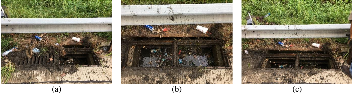
Figure B.49: BUCHER RECycler 315 Operations on September 26, 2018 in Franklin County (a, b) Structure prior to cleaning, (c) Structure post cleaning.
