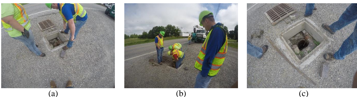
Figure B.3: VJT Operations Using Vac-Con 9CY on June 25, 2018 in Union County (a) Structure prior to cleaning, (b) Cleaning of the structure, (c) Structure post-cleaning.
