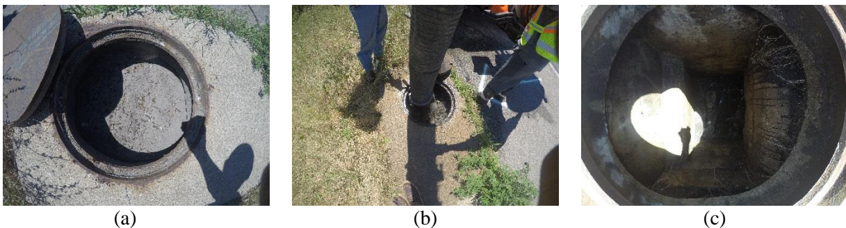
Figure B.36: VJT Operations Using Vactor 2100 on July 17, 2018 in Franklin County (a) Structure prior to cleaning, (b) Cleaning of the structure, (c) Structure post cleaning.
