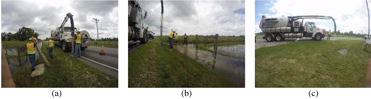
Figure B.13: VJT Operations Using Vactor 2100 on June 27, 2018 in Union County (a) Zone setup, (b) Cleaning of the structure, (c) Zone breakdown.
