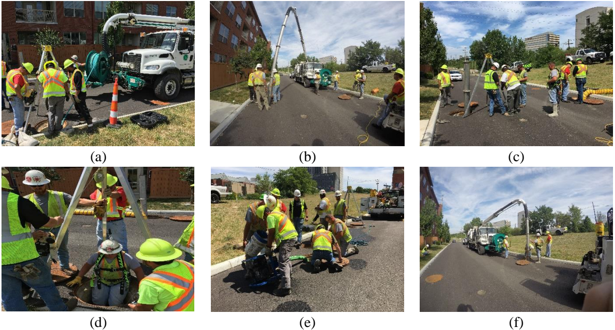
Figure 6.4: Hydrodynamic Separator Maintenance Using Traditional VJT Methods. (a, b) VJT cleaning junction chamber so that crew member may be sent in to plug upstream line, (c) Crew waiting for junction chamber air to circulate and achieve acceptable oxygen and gas levels, (d) Crew member lowering into junction chamber to plug upstream line with sandbag, (e) Crew setting up a pump to remove standing water from hydrodynamic separator, (f) VJT cleaning the hydrodynamic separator.
