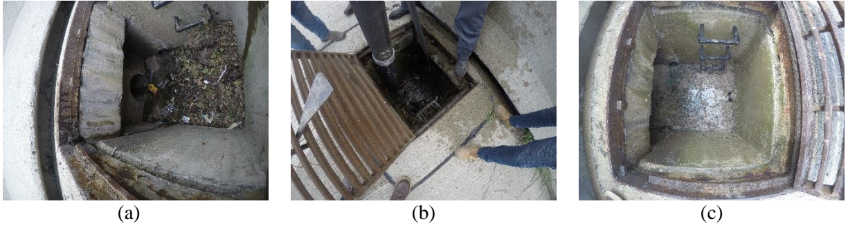
Figure B.29: BUCHER RECycler 315 Operations on July 16, 2018 in Franklin County (a) Structure prior to cleaning, (b) Cleaning and jetting of the structure, (c) Structure post cleaning.
