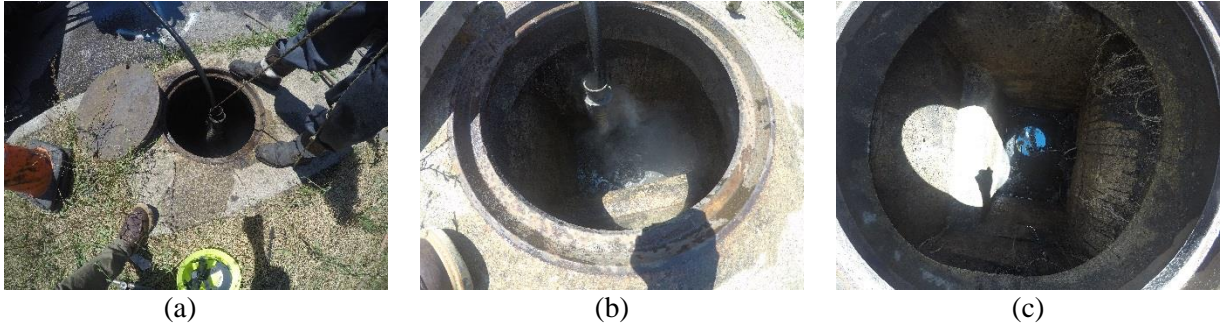
Figure B.37: VJT Operations Using Vector 2100 on July 17, 2018 in Franklin County (a, b) Jetting the underdrain of the structure, (c) Structure cavity post jetting.
