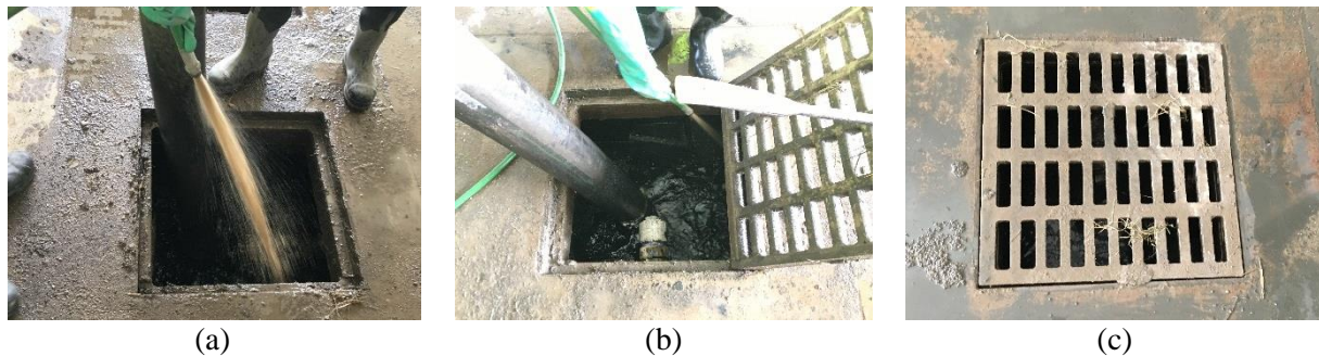
Figure B.68: BUCHER RECyler Operations on October 11, 2018 at ODOT West Jefferson Garage (a, b) Running vacuum and small hose on the structure, (c) After cleaning the structure.
