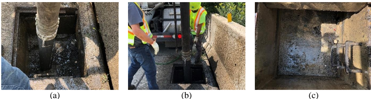
Figure B.44: BUCHER RECYcler 315 Operations on August 22, 2018 in Franklin County (a) Cleaning the structure, (b) Operators cleaning and spraying debris with small hose, (c) Post cleaning.
