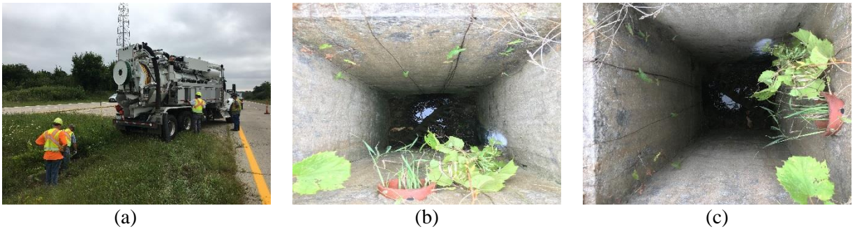
Figure B.46: BUCHER RECycler 315 Operations on August 30, 2018 in Madison County (a) Operators setting up zone, (b) Structure pre-cleaning, (c) Structure post cleaning.
