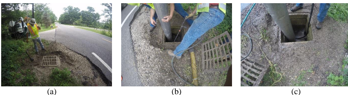
Figure B.2: VJT Operations Using Vac-Con 9CY on June 25, 2018 in Union County (a) Structure prior to cleaning, (b) Cleaning of the structure, (c) Jetting through structure line.
