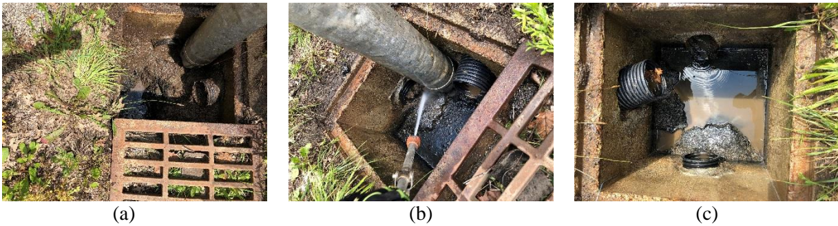
Figure B.14: VJT Operations Using Vactor 2100 on June 28, 2018 at ODOT Richwood Garage (a, b, c) Structure during cleaning.
