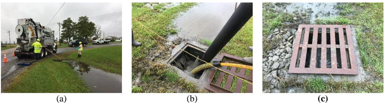
Figure B.48: BUCHER RECycler 315 Operations on September 25, 2018 in Union County (a) Operators setting up zone., (b) Cleaning of the structure, (c) Structure post cleaning
