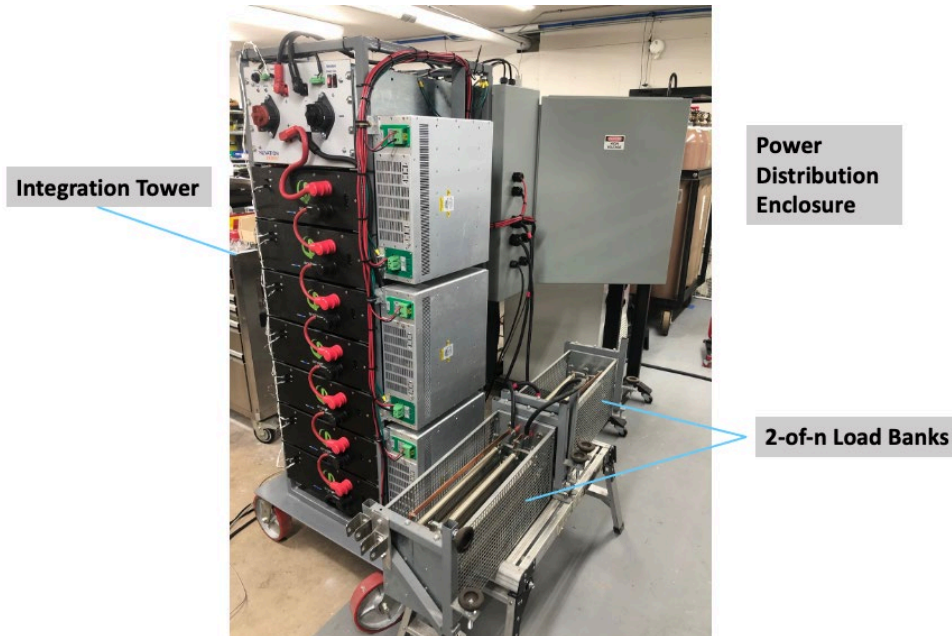
Figure 28. Integration tower and load banks simulating locomotive DC loads
