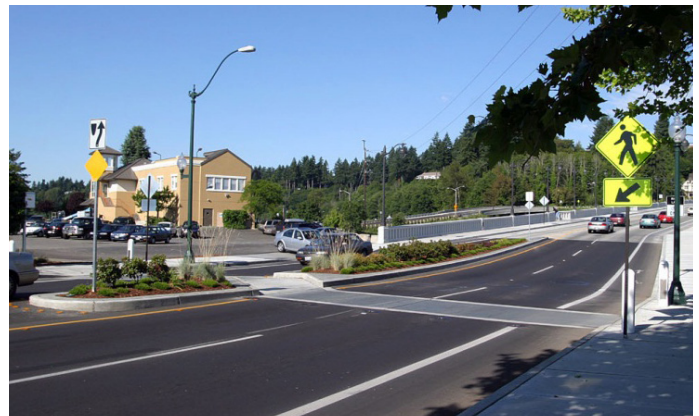
Figure 1. Pedestrian refuge island on four-lane road in south Florida. 1
