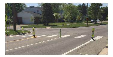
Figure 2. Gateway configuration of the R1-6 in-street sign with a reflective delineator on the lane markings. Location: Nixon Road at Bluett Road, Ann Arbor, MI.<sup>1</sup>
