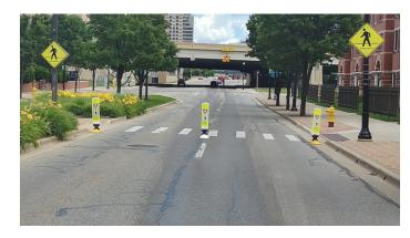
Figure 1. Gateway configuration of the R1-6 In-Street Pedestrian Crossing sign with two lanes in the same direction.<sup>1</sup>
