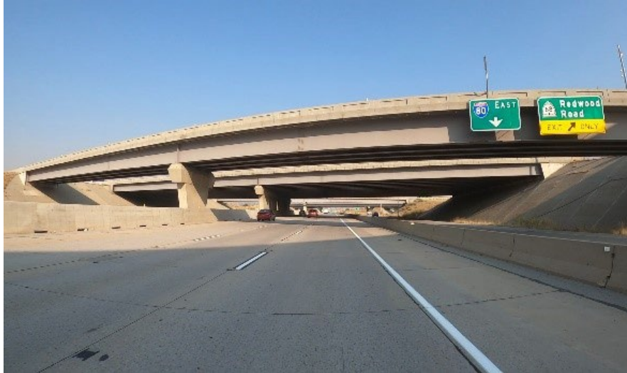
Figure 5.9 The target bridge
